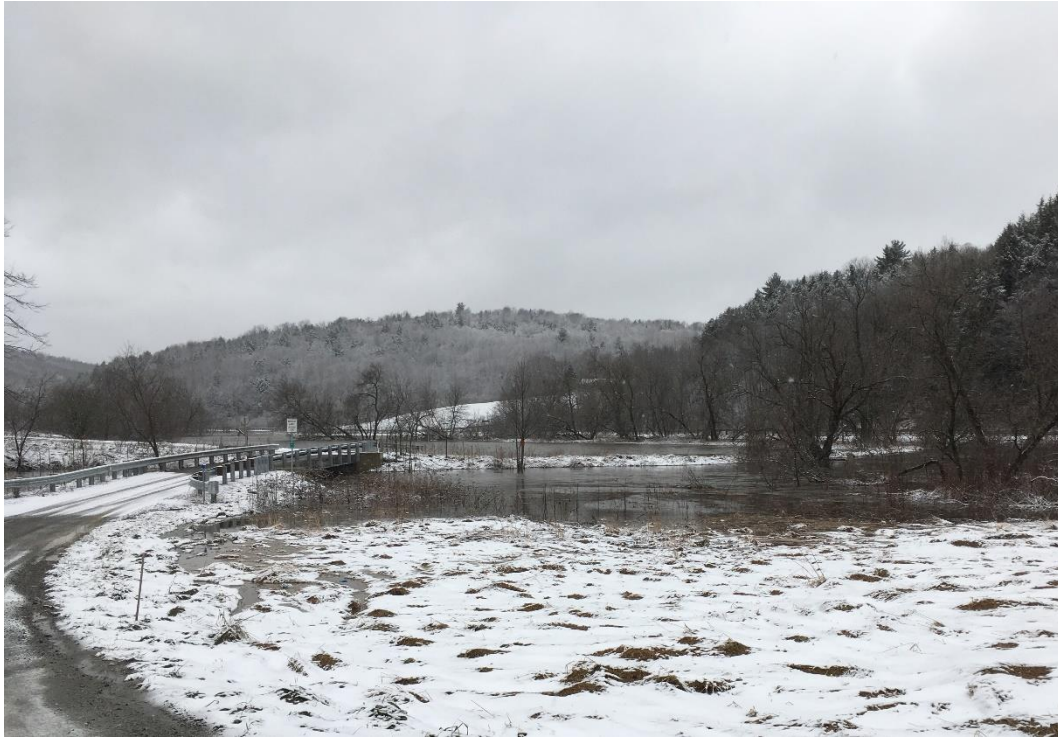
View to bridge outlet from Jct of Elm Brook Rd and VT Route 36, 12/22/2018
