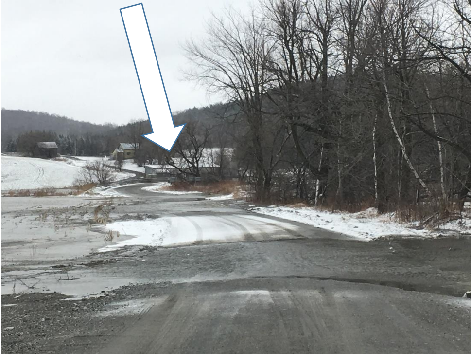
View to northeast from VT Route 36 down Brusso Rd, bridge at arrow, 12/22/2018
