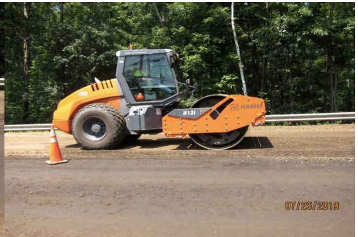
(h) Smooth drum compactor following road grader
