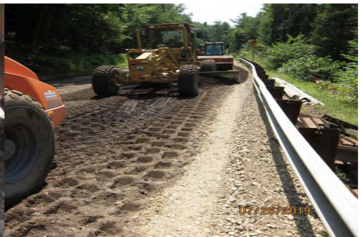
(f) Road grader and smooth drum compactor following sheep's foot compactor
