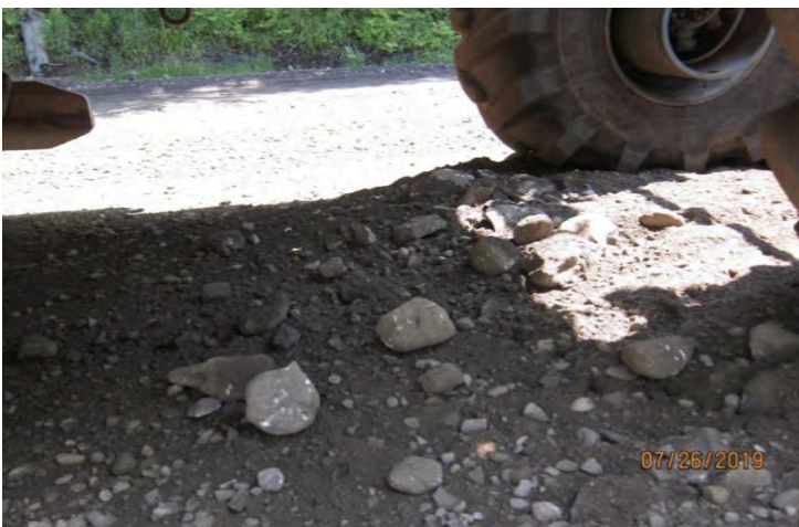
(e) Typical base composition behind grinding/mixing drum
