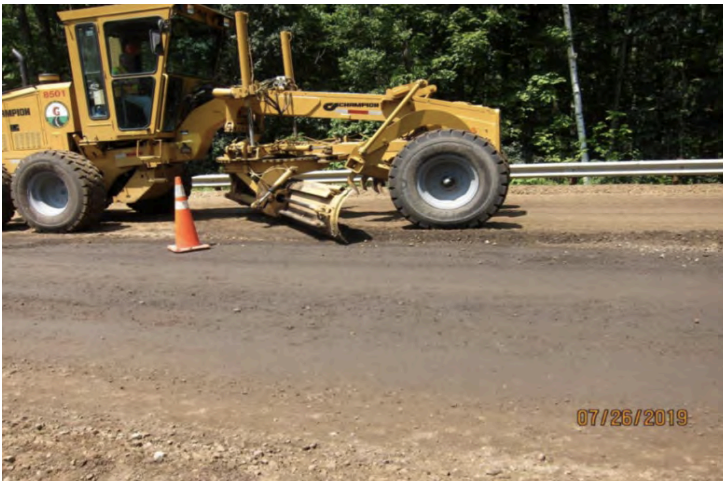
(g) Road grader fine grading base following grinding/mixing train
