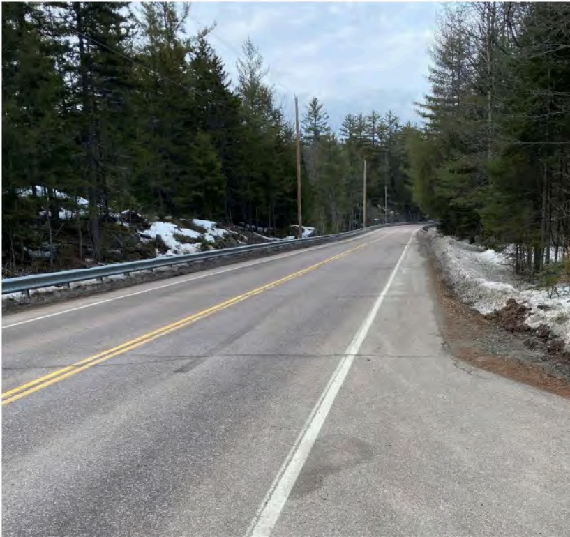
(c) Vermont 12 Worcester-Elmore at southern portion on March 12, 2020
