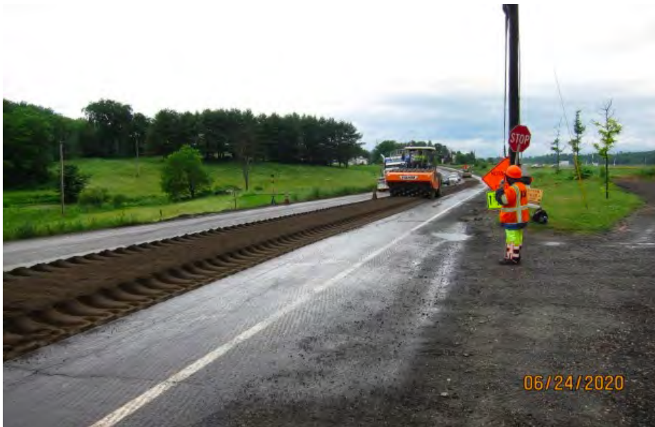
(d) Sheepfoot compactor following reclaimer, with smooth drum roller behind
