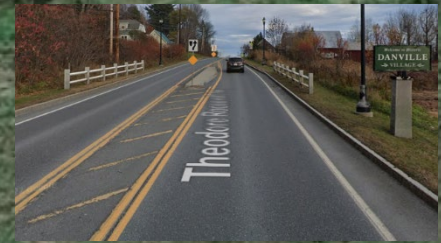
Lateral shift along US-2 entering Danville, Vermont
