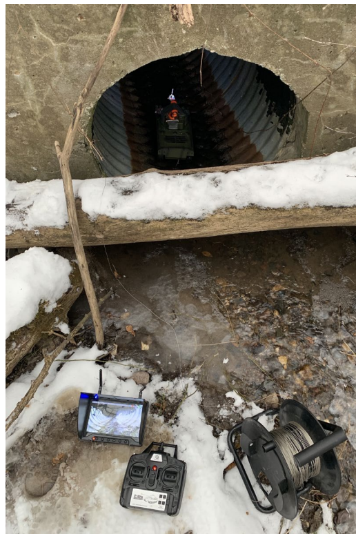
Figure 17 Mobility testing of HIVE 2.0 Tank in metal lined culvert with flowing water and separation gap in Culvert 64099 under U.S. Route 7 in Charlotte, VT
