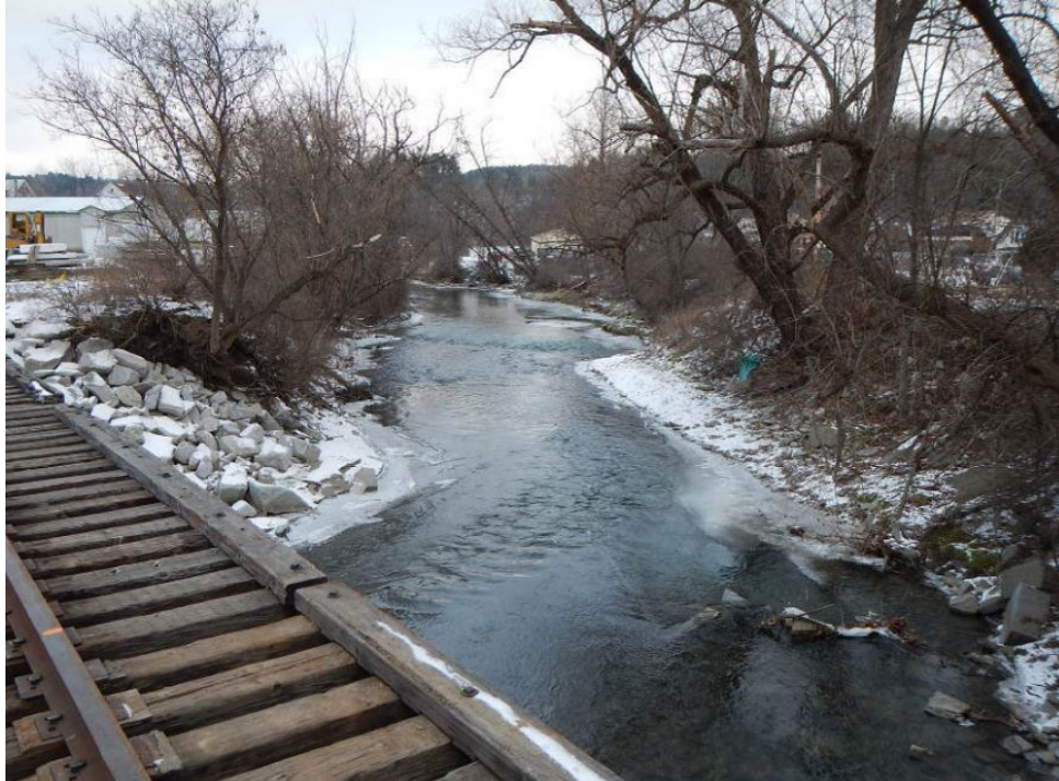
Looking downstream at Stevens Branch from Bridge 308
