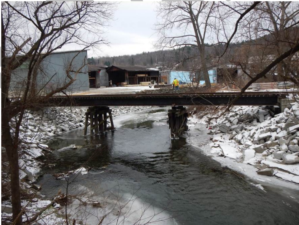
Looking upstream along Stevens Branch at Bridge 308
