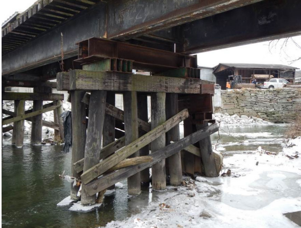
Looking at Pier 1 from west bank
