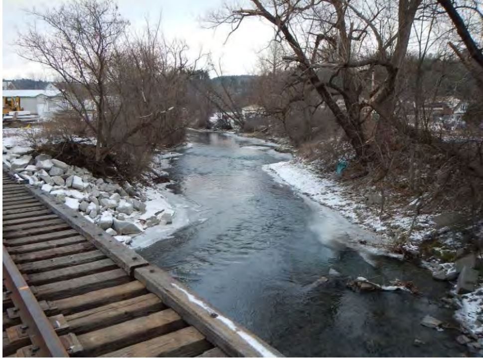
Looking downstream at Stevens Branch from Bridge 308
