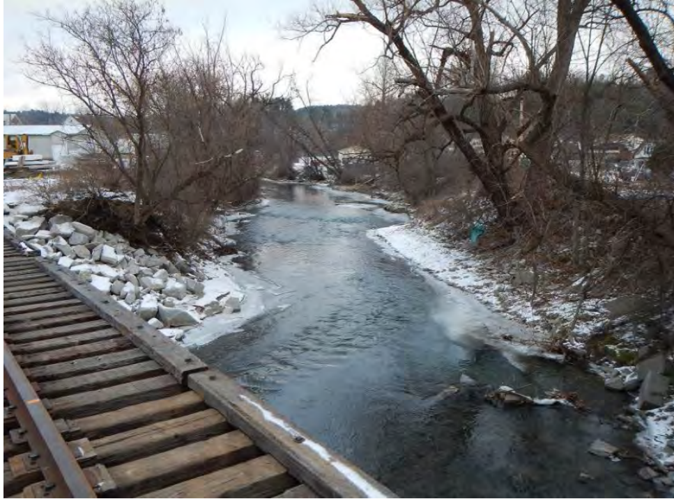
Looking downstream at Stevens Branch from Bridge 308
