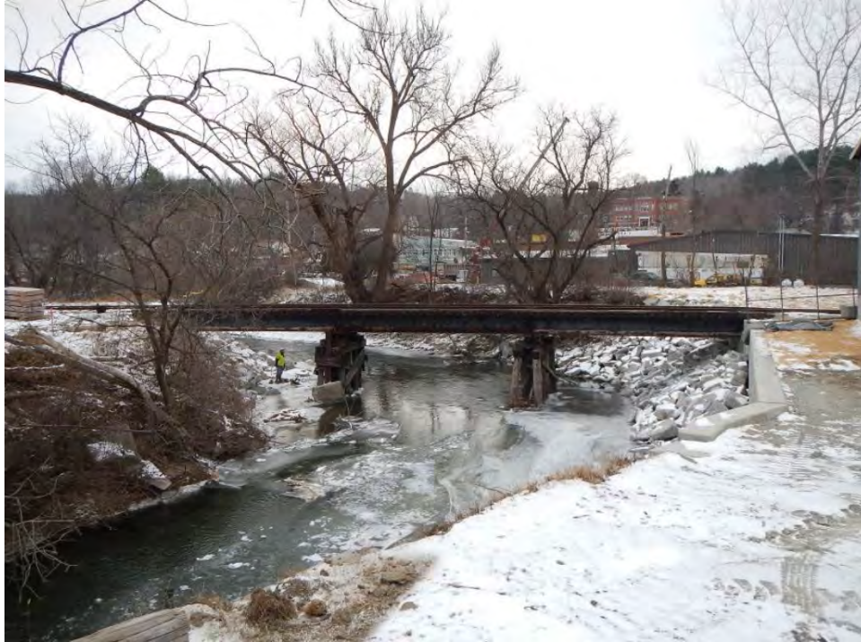
Looking downstream along Stevens Branch at Bridge 308
