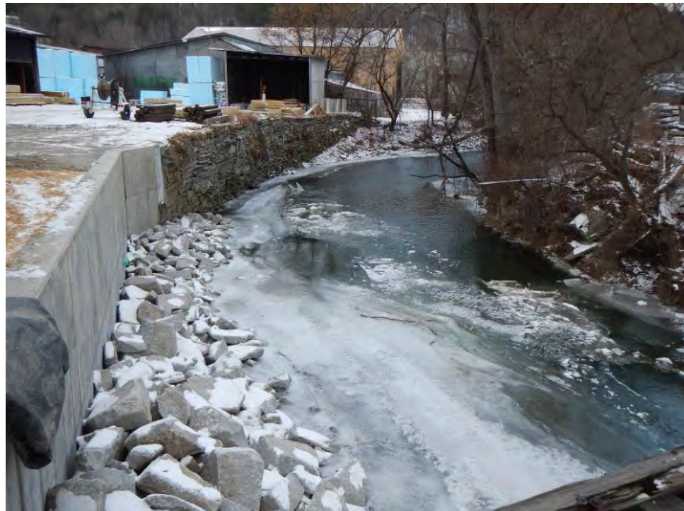
Looking upstream at Stevens Branch from Bridge 308
