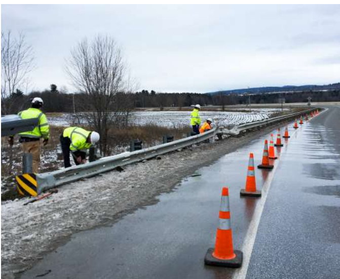
SHELDON. While the cold can be challenging, VTrans crews do as many tasks as winter weather allows. A brief mid-season snow melt enabled crews to take care of badly damaged guardrail along VT-105.
