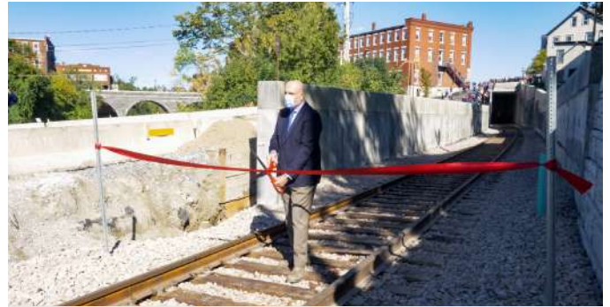
MIDDLEBURY. After many months of excavation and construction, the new rail tunnel in Middlebury officially opened on September 18, 2020. People gathered to witness the first passenger train pass through the tunnel and congregated on Main Street as roads through the downtown were officially reopened.
