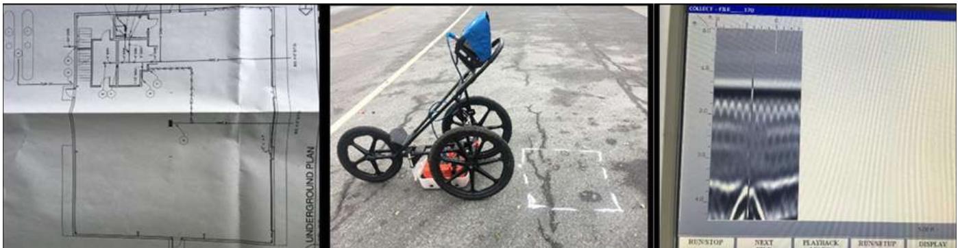
NEWPORT. The GPR being used at Northeast Kingdom International Airport to confirm the presence and precise location and depth of a floor-drain outlet pipe exiting a hangar and being used at a gas station to locate a drop inlet previously paved over.
