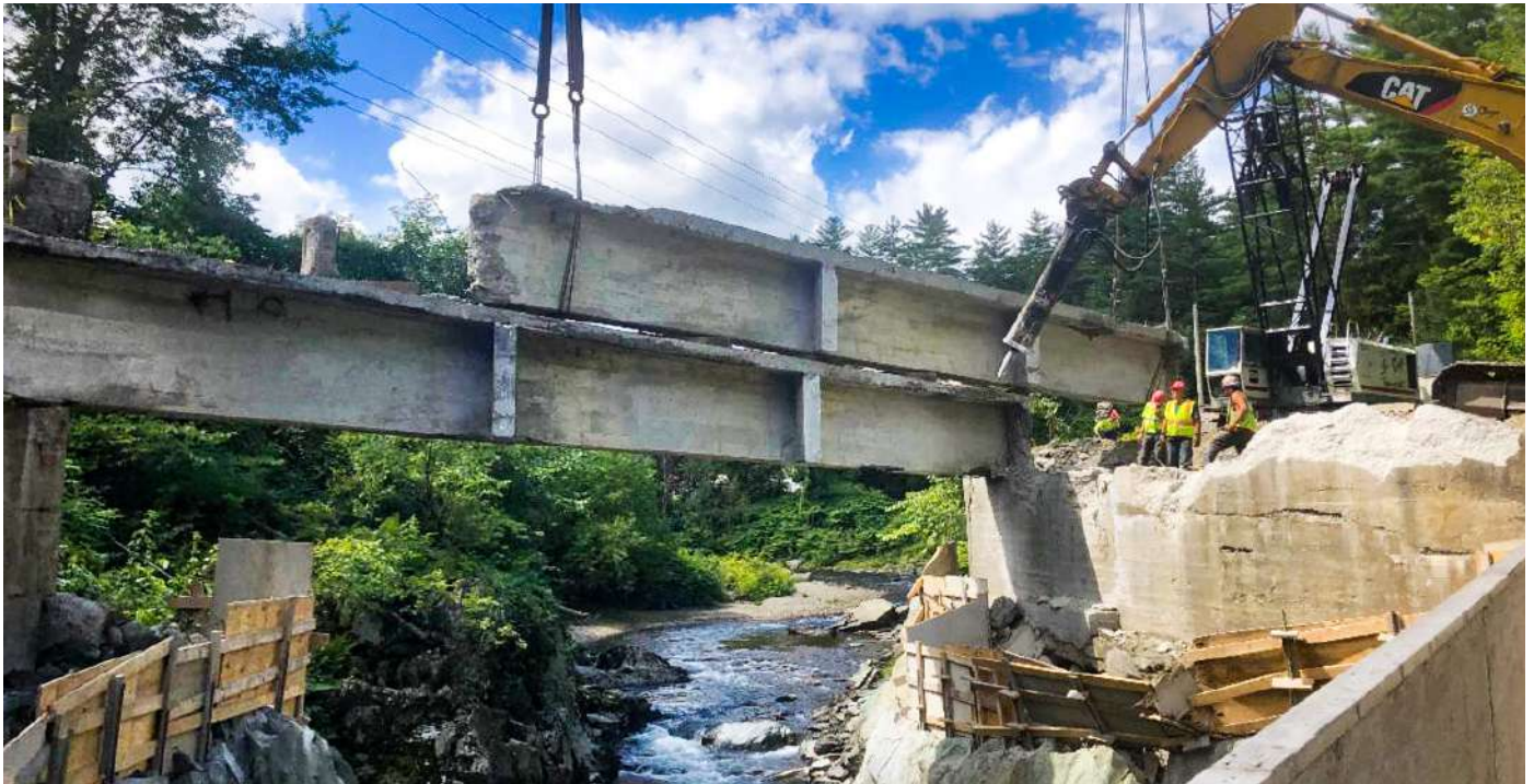
MORETOWN. Built in the 1920s, the original concrete bridge spanning the Mad River along VT-100B was badly in need of replacement. A two-month closure period allowed the old bridge to be demolished quickly, with a new bridge built on a slightly modified alignment. The new structure now spans 100 feet and features wider lanes and shoulders for a safer traveling experience for all.
