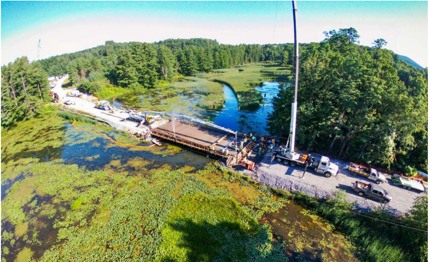
GEORGIA. The replacement of a narrow bridge along VT-104A demonstrated how good planning can rapidly accelerate the construction process. Within the first day of closing the old bridge, the original deck was removed, preparations for the new foundation had begun, and new steel girders arrived on site. Working fast, the project team was able to open the new bridge to traffic within just 37 days.
