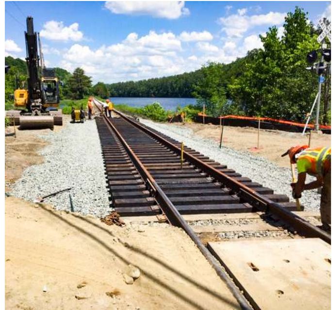
NORWICH. Pictured above is a railroad crossing reconstruction project along River Road in Norwich. The project saw the replacement of concrete surface panels, rail ties, rail ballasts, and the addition of a new active warning signal system with LED lights.
