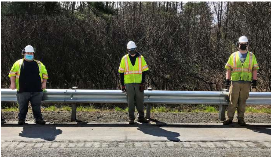
THETFORD. As many students transitioned to online learning, VTrans Intern Maintenance Workers were getting valuable on-the-job experience. Interns from our Thetford garage learned how to repair a damaged guardrail, while social distancing and following safety protocols.
