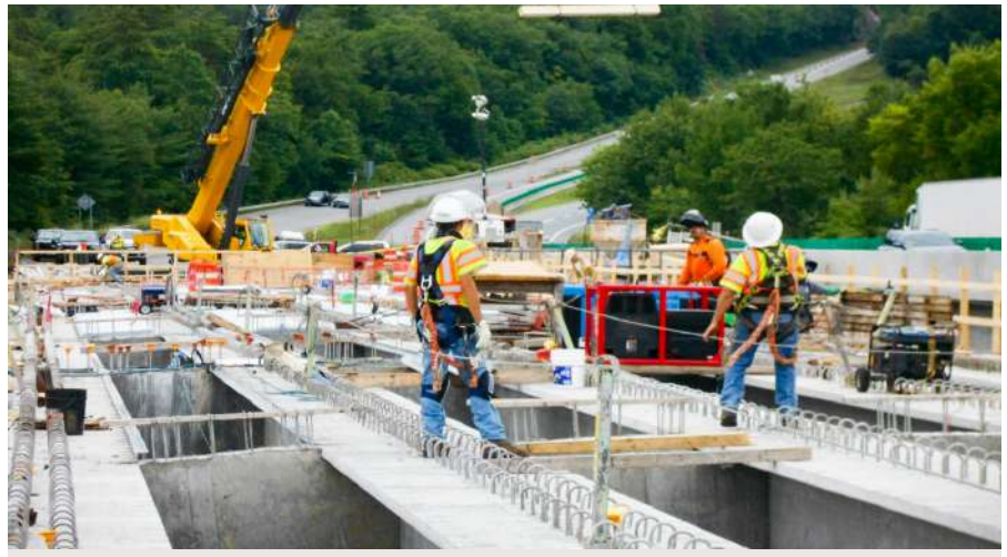
ROCKINGHAM. The multi-year bridge replacement project along I-91 continued in 2020, with the main focus on the building of the new bridge decks. These two new bridges will ultimately feature wider lanes, ensuring safer travel for all.
