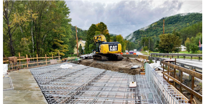
CHESTER. A multi-year bridge replacement project began along VT Route 103 in Spring 2022. The bridge deck has been replaced and minor repairs were made to the bridge piers, beams, and bearings. Crews will return in Spring 2023 to complete work on expansion joints, landscaping, and punch list items.
