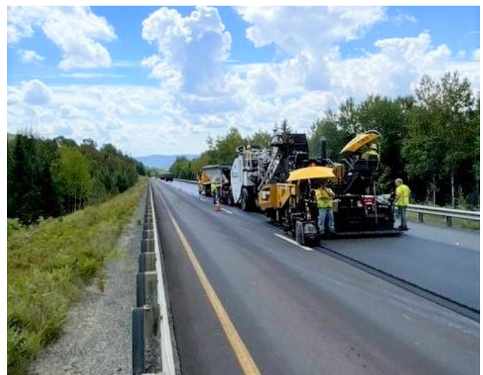
LYNDON-BARTON. A 40-mile interstate paving project began along I-91. Spanning three exits, work will also include guardrail replacement and drainage improvements.
