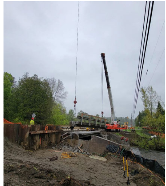
CALAIS. A series of bridge replacements continued on VT Route 14. With Bridge 74 completed in 2021, work began on Bridge 77 and Bridge 82, both over the Kingsbury Branch of the Winooski River. Originally built in the 1910s-1920s, all three bridges required significant work to be brought up to modern standards. Bridges 74 and 82 were completely replaced, while Bridge 77 underwent a deck and superstructure replacement but kept the existing substructures due to its better condition. The new expected service life of Bridges 74 and 82 is now 75 years, with the the superstructure of Bridge 77 projected at 40 years.
