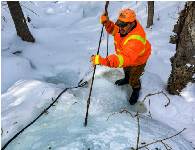
WARRENS GORE. In addition to affecting road surfaces, cold snaps and extreme winter weather can impact infrastructure under the roadway. Maintenance crews are tasked with keeping culverts unobstructed, which sometimes necessitates thawing a frozen culvert.
