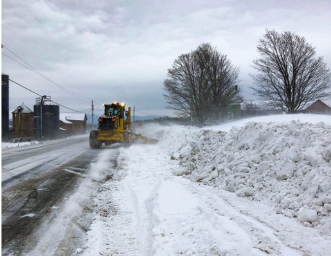
FRANKLIN. Even after a winter storm is over and snowplows have cleared a roadway, our maintenance crews stay busy. A crew pushed back snowdrifts caused by wind gusts along VT Route 120.
