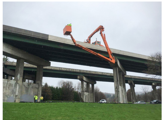
SPRINGFIELD. Proper “basket training” is essential for VTrans staff to properly inspect many of the bridges in our highway network.
