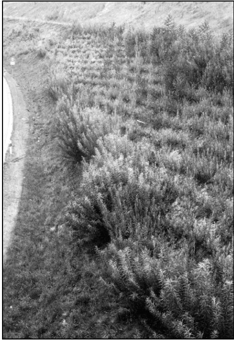
Shrubs used for stabilizing a slope planted in grid pattern.
