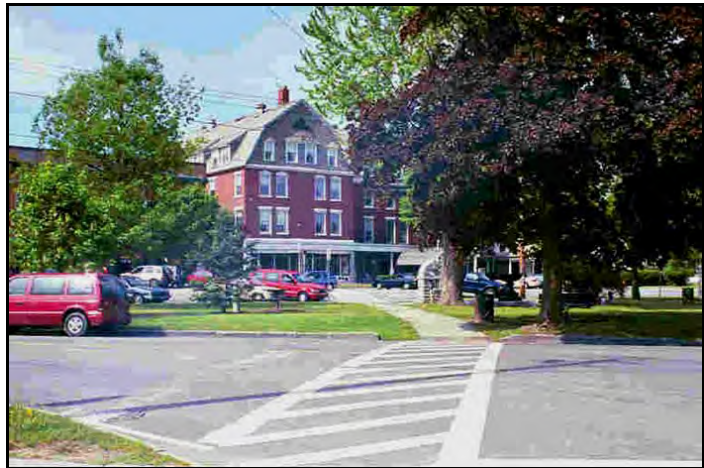
It may be possible to save important trees by adjusting the roadway alignment in the early phases of the project. This photo shows Route 7 and the green in Brandon in front of the Brandon Inn.
