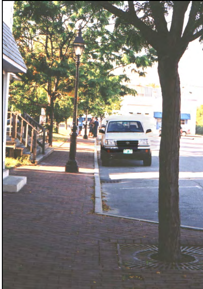
Planted curb extension island on a local road in Essex Junction protects parked cars and improves the roadway crossing for pedestrians.
