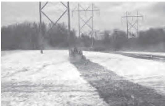
Incorporating lime to adjust soil pH prior to making a native grass planting at Londonderry, NH,
