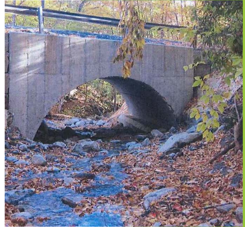
New bridge, Duxbury
