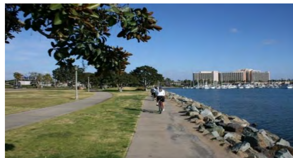
Figure 3: Bikeway (Concrete Bicycle Path)
