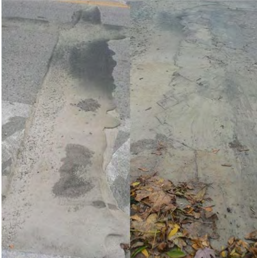
Figure 8 Side by side comparison of an overfilled joint (left) and the same joint after removal of material (right)
