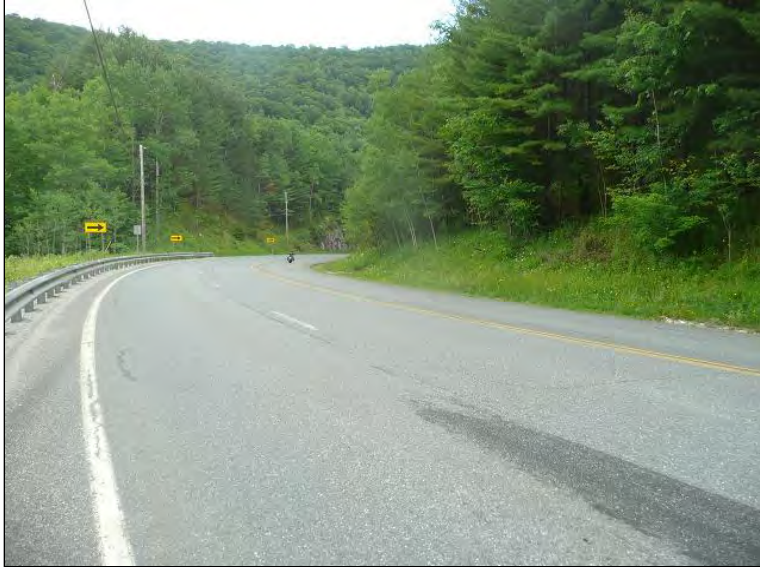
Figure 11: Overview of site
