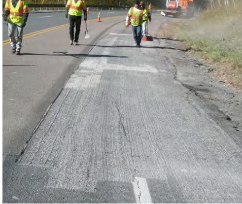
Figure 6: Repair area, after grinding and sweeping
