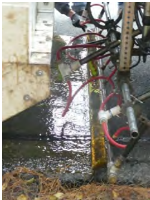
Figure 2: Epoxy truck application
