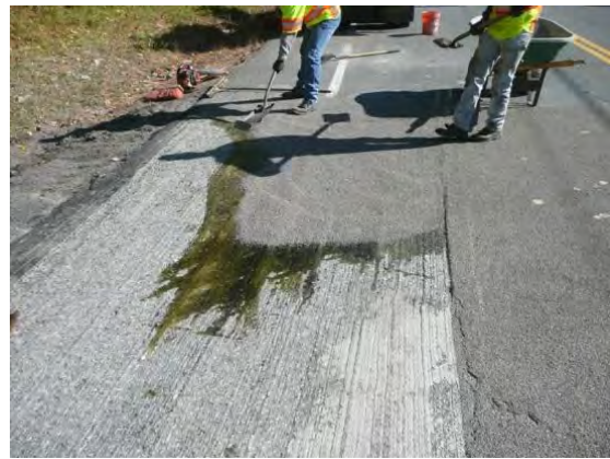
Figure 9: Spreading the aggregate
