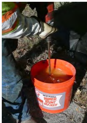
Figure 7: Mixing the epoxy
