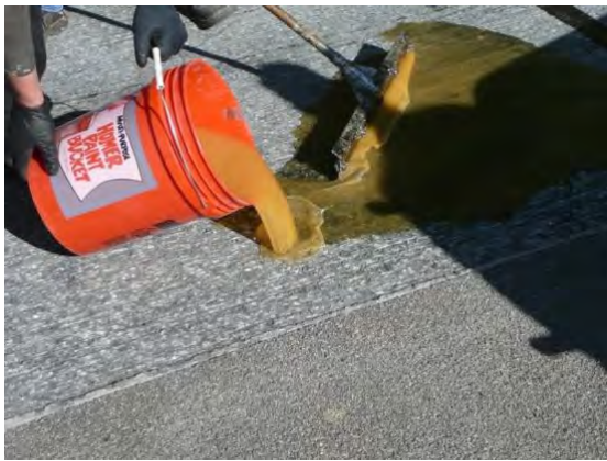
Figure 8: Pouring the epoxy
