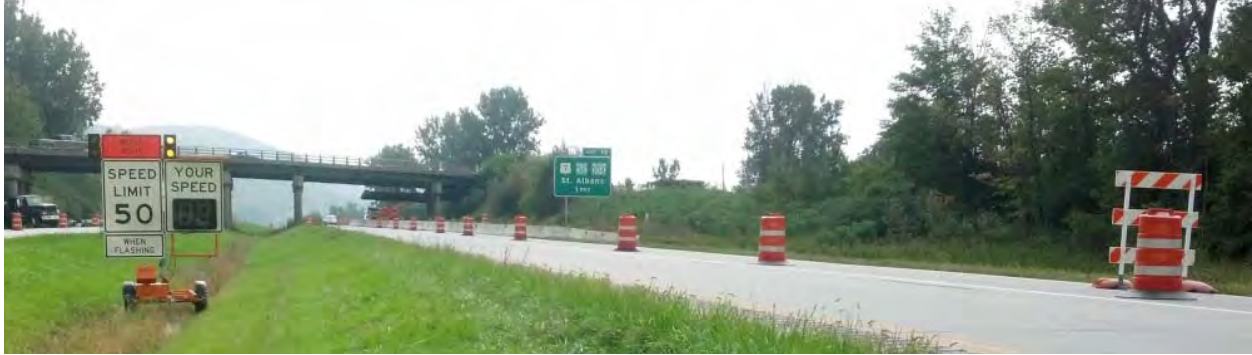
Figure 7 Saint Albans Bridge 90, Northbound RSFS
