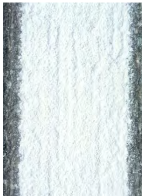
Figure 8: Test Site 5, White Skip Line
