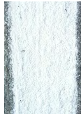
Figure 9: Test Site 5, White Edge Line
