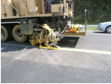
Figure 2: Spray Application of Northbound Yellow Line Delineation
