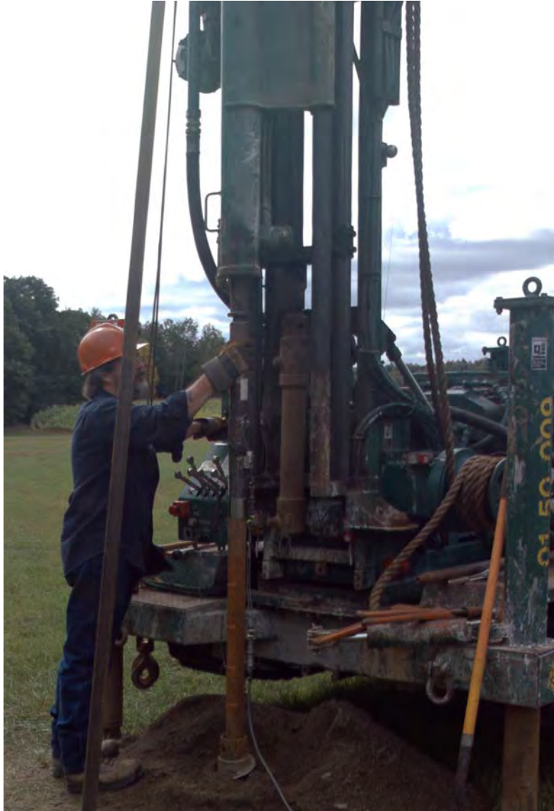
Figure 9 Placing Automatic Hammer on top of Drill String.
