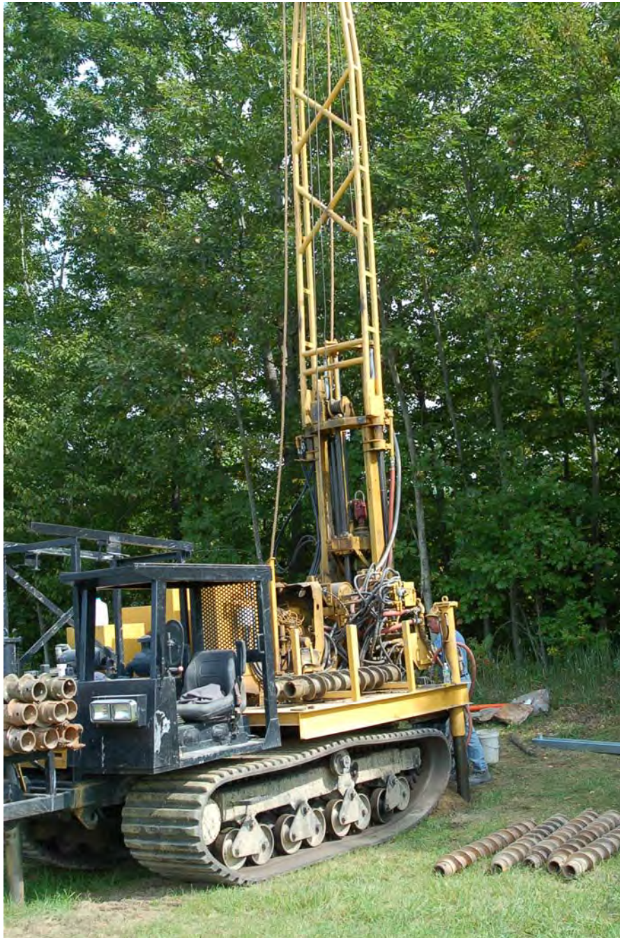
Figure 4 TransTech CME 75 on Track Rig used for Boreholes GD-5 and GD-6.
