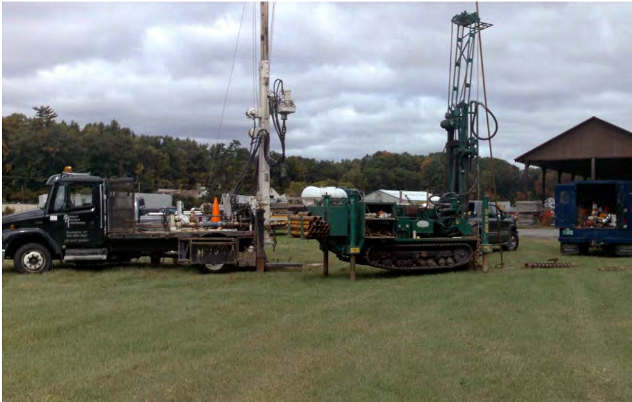
Figure 15 Photo of Test Site while Drilling Boreholes GD-8 and GD-9.
