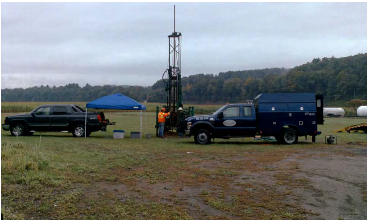
Figure 14 Photo of the Test Site at Borehole GD-8.
