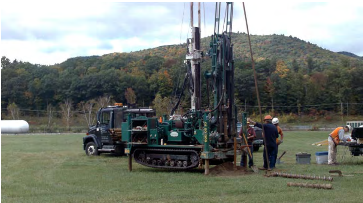
Figure 3 VTrans CME45C on Track Rig used for Boreholes GD-7 and GD-8.
