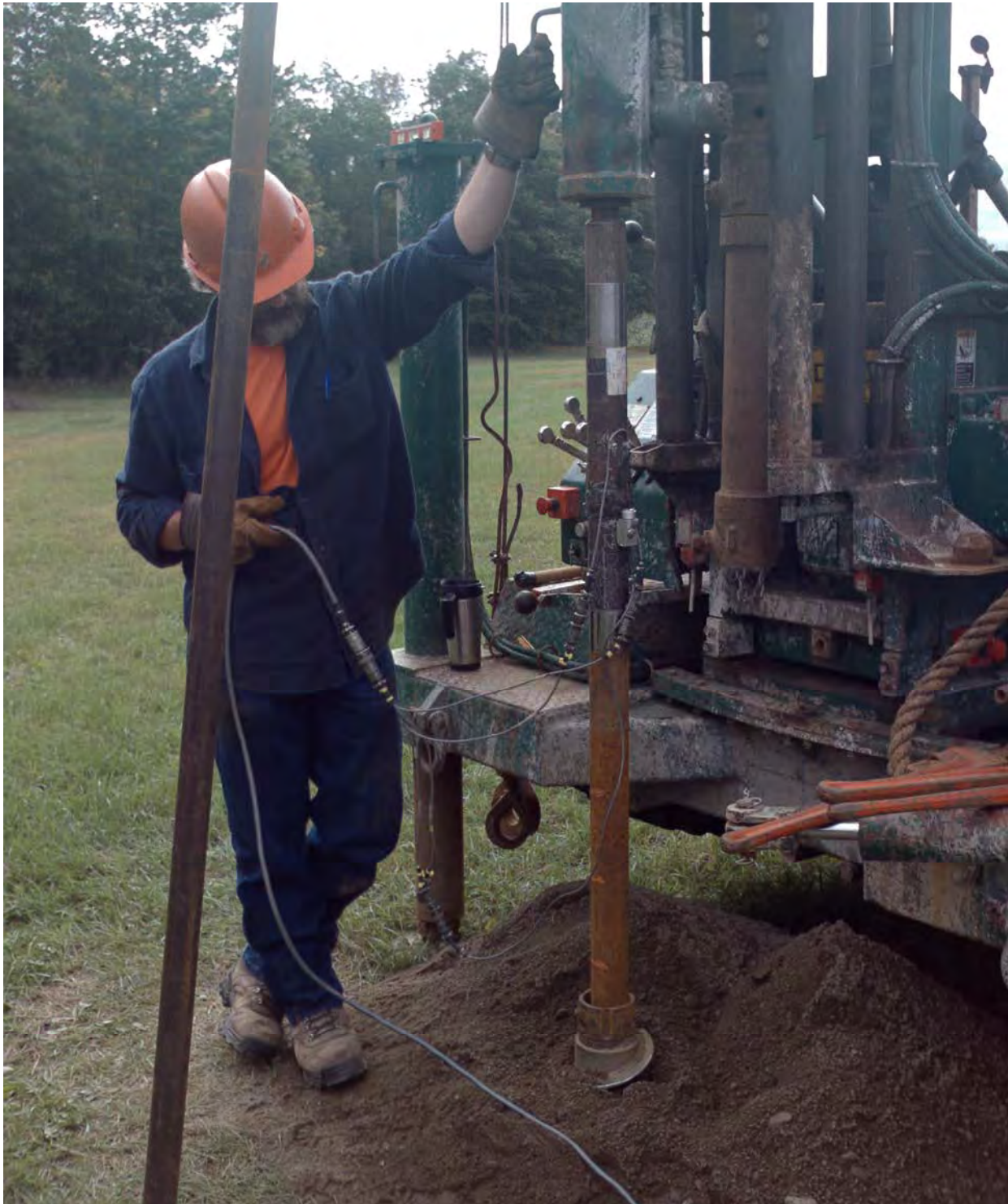
Figure 11 NWJ Instrumented Drill Rod with Driller Holding Wires During Driving.
