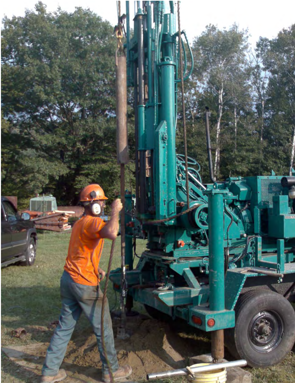
Figure 7 Photograph of Safety Hammer with Driller “Throwing the Rope” at GD-4.
