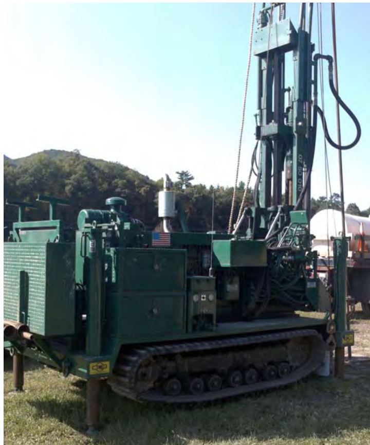
Figure 1 VTrans CME 55 used on Boreholes GD-1 and GD-3.
