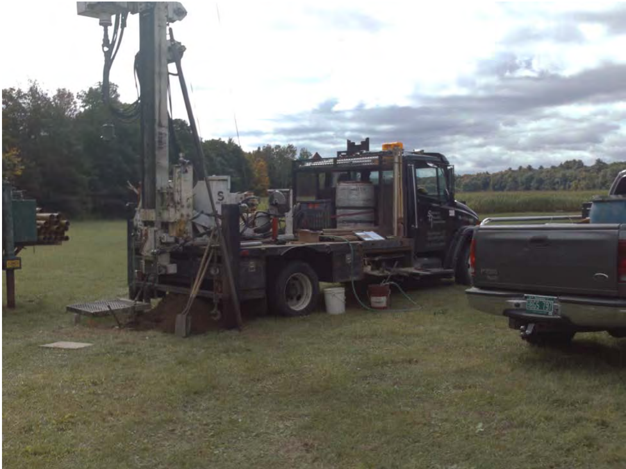
Figure 5 SDI Simco Drill Rig used for Borehole GD-9.
