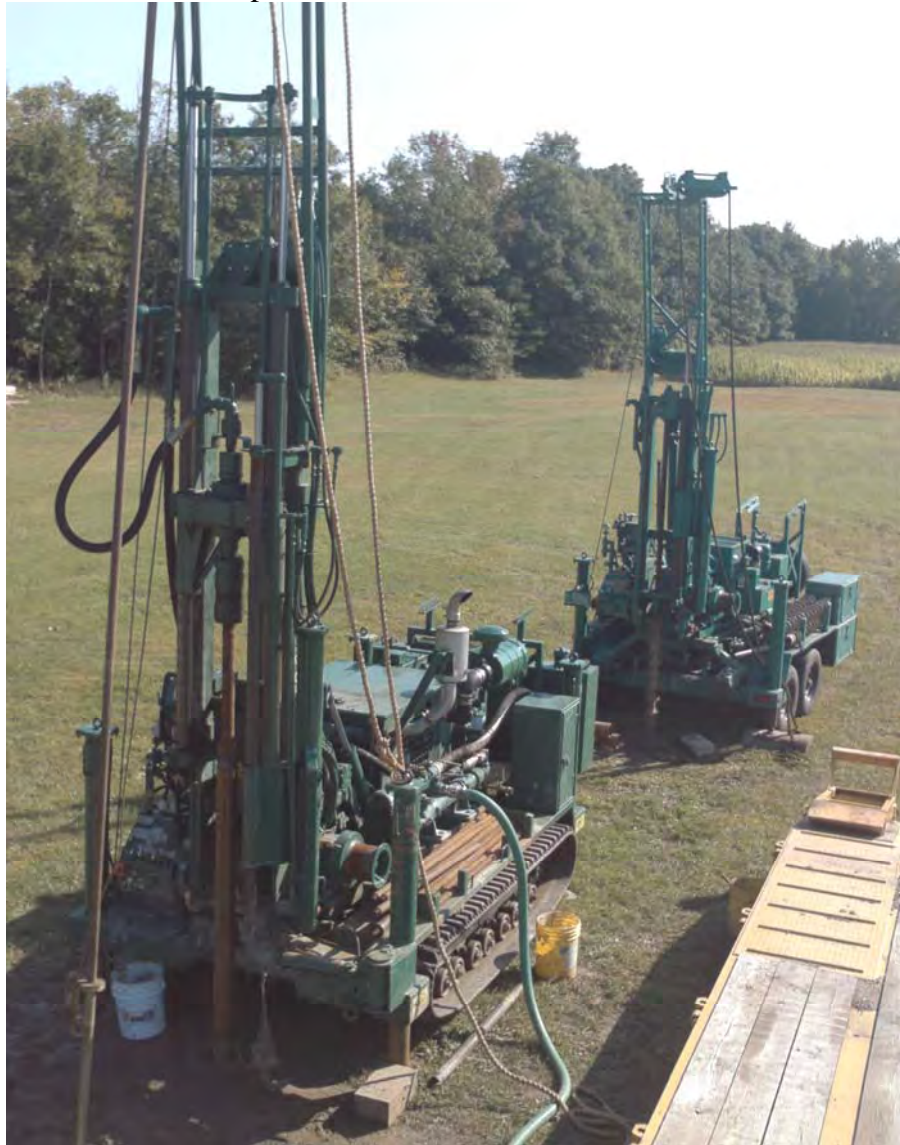
Figure 6 Drill Rigs using HSA and Washed Bore Drilling Techniques.
