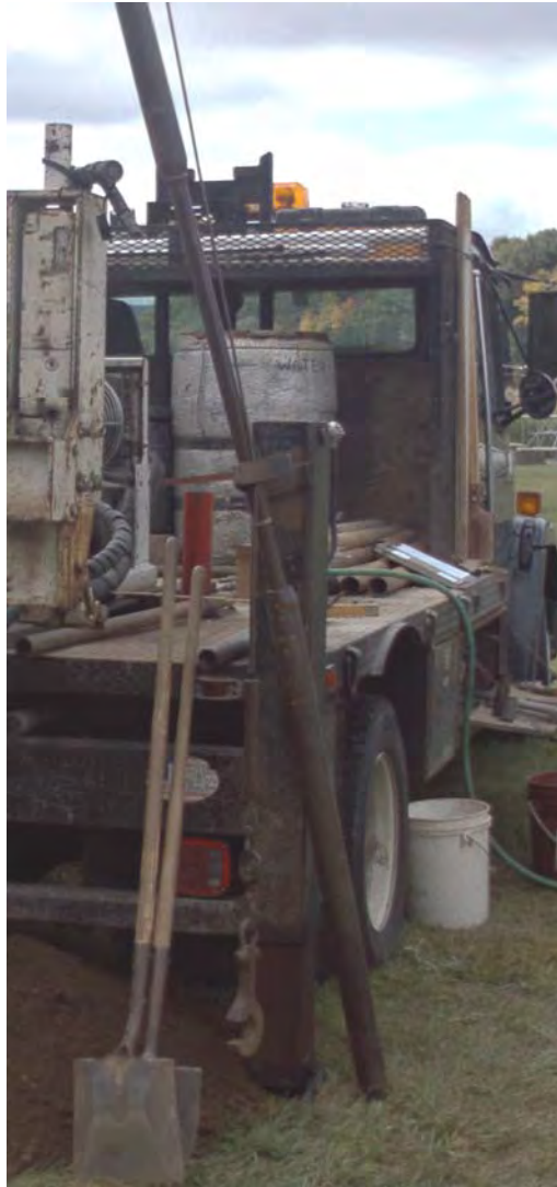
Figure 8 Photograph of Down-Hole Safety Hammer (leaning on right hand side of rig).
