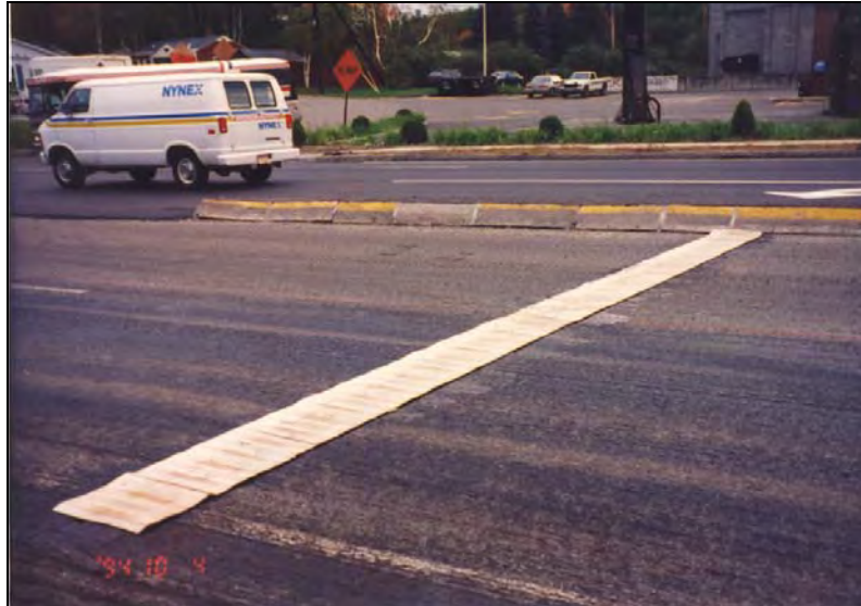
Figure 8 – Hartford PavePrep Installation
