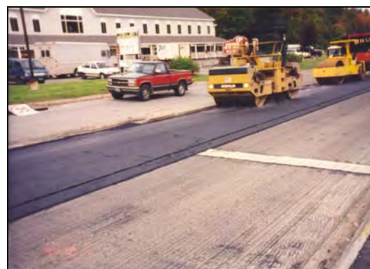
Figure 10 – Hartford Paving Overlay
