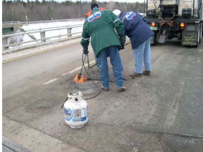
Figure 1: Surface Preparation
