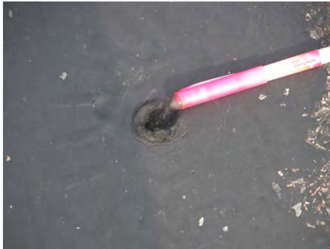
Figure 3: Displacing the Pot Hole Patch Material
