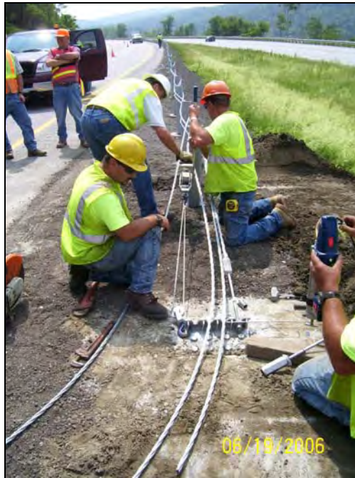
Figure 1 – Brifen Wire Rope Installation
