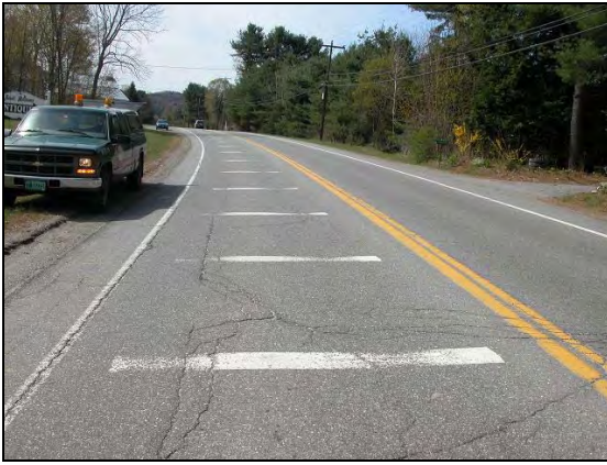
Figure 6 – South Side of Newfane Village
