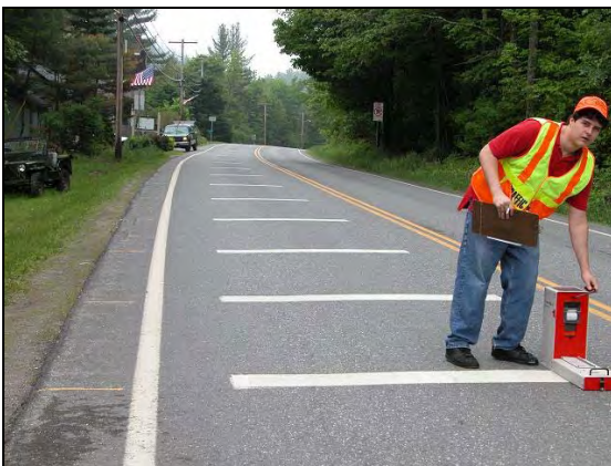
Figure 8 – South Side of Townshend
