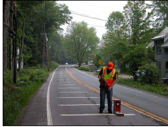
Figure 7 – North side of Newfane Village
