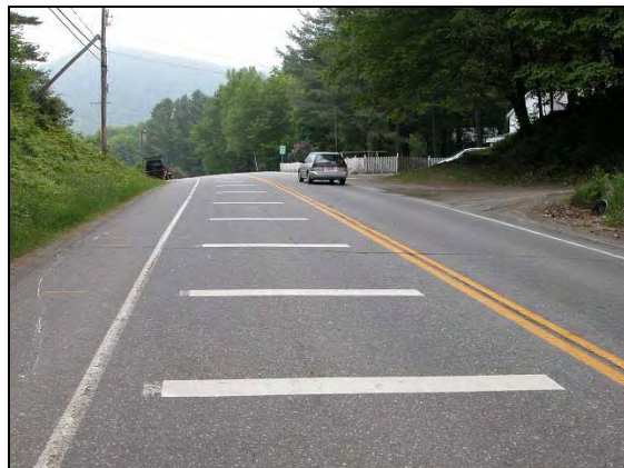
Figure 9 – North Side of Townshend
