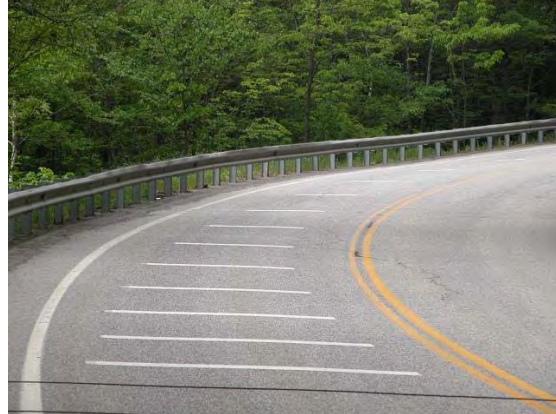
Figure 11 – North Side of Townshend
