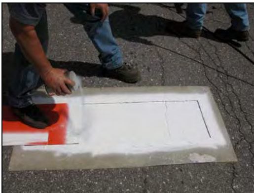
Figure 4 – Application of Glass Beads
