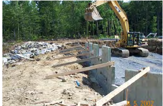
Figure 4: Placement of first row of panels
