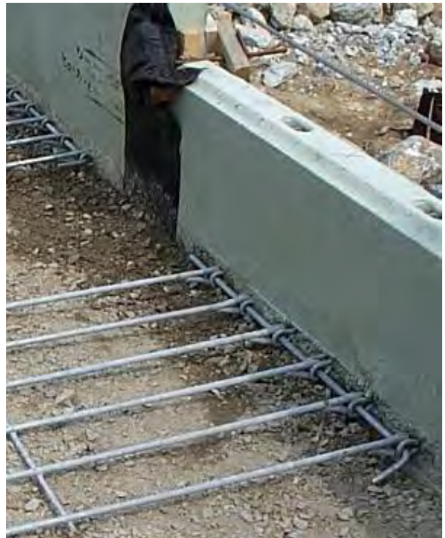
Figure 5: Reinforcement Mesh Attachment to Panel
