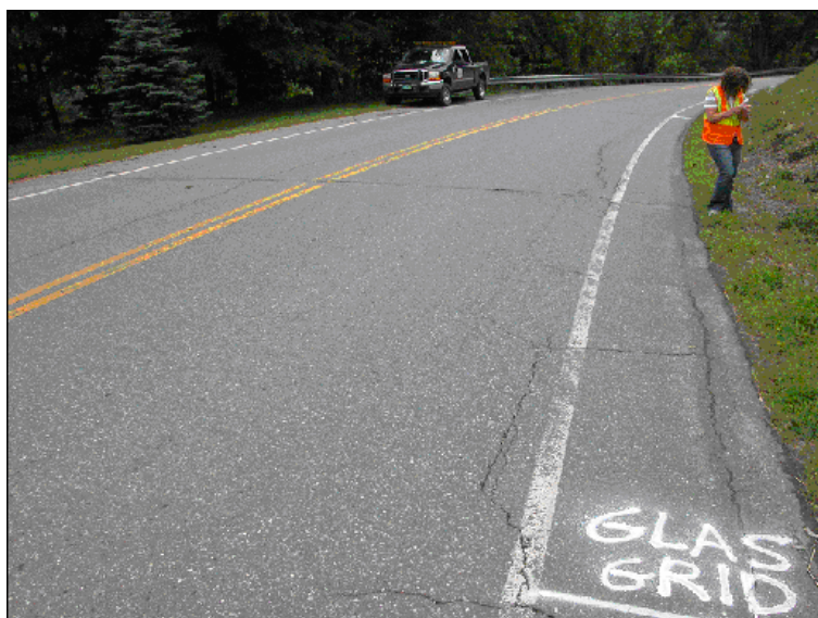
Figure 10 – Southbound view of Barnett test site in 2007
