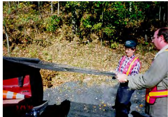
Figure 6 – Installation in Barnet
