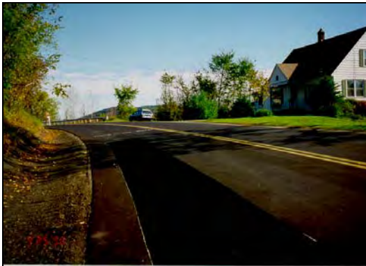
Figure 5 - GlasGrid Placement in Barnet
