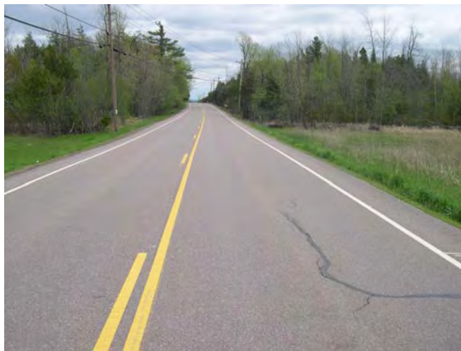
Figure 7 -VT 314 Grand Isle (2000) Test Site 2
