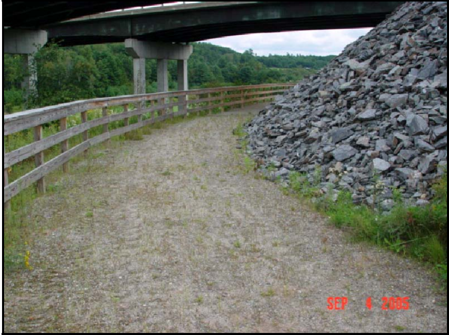
Figure 43: Cross Vermont Trail - Safety Railing
