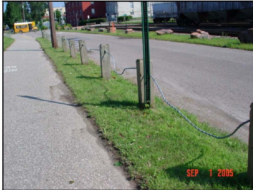
Figure 40: Burlington - Cable Fencing
