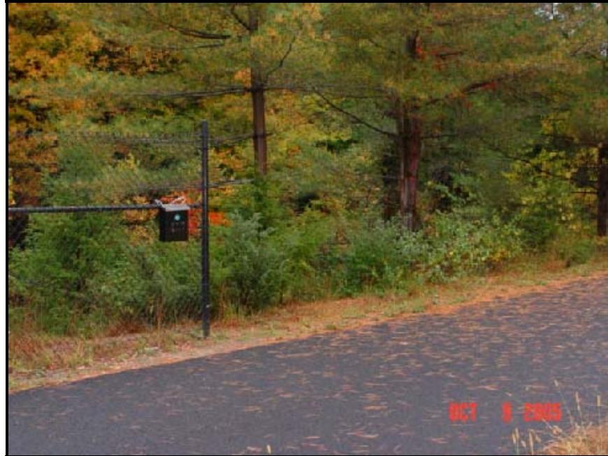
Figure 55: Toonerville - Inconsistent Use of Fencing
