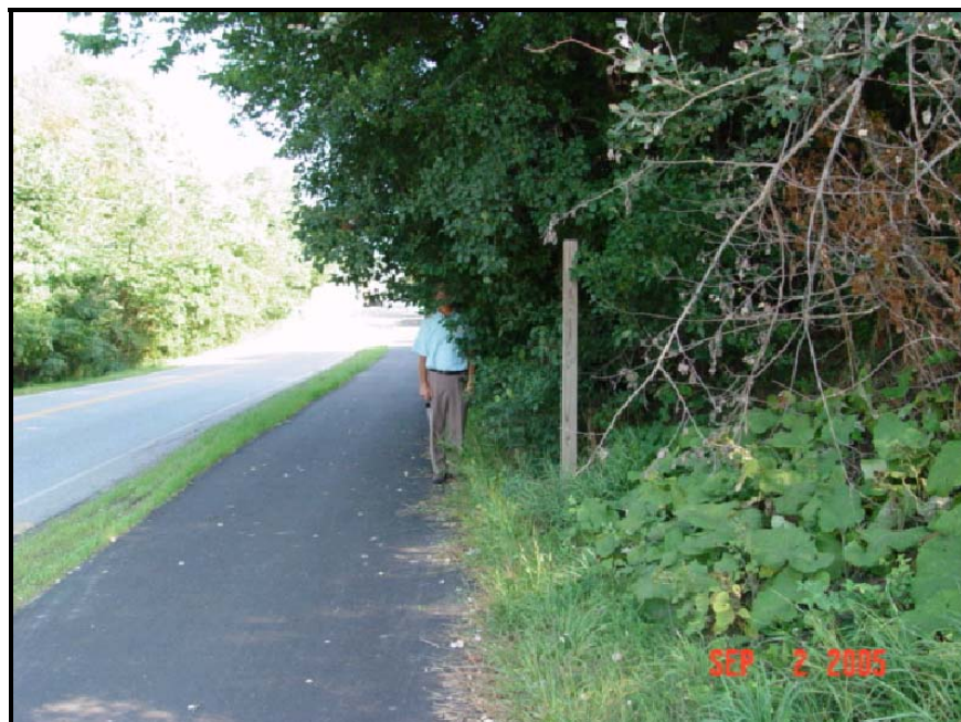
Figure 35: South Burlington - Potential Vegetation Overgrowth
