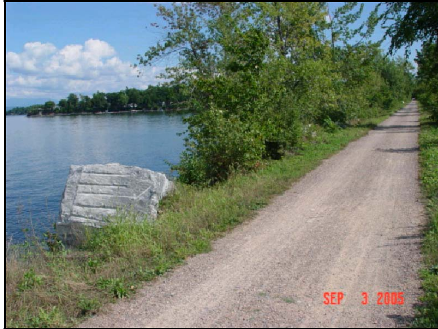
Figure 31: Colchester Causeway - Boulders at Water Body
