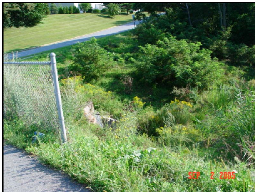
Figure 54: South Burlington - Inconsistent Use of Fencing
