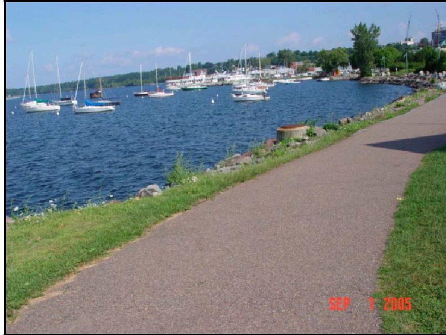
Figure 27: Burlington Waterfront - No Clear Zone to Potentially Hazardous Water Body
