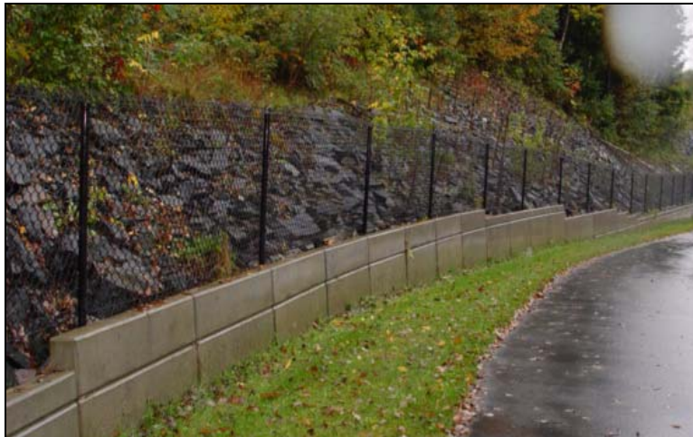
Figure 23: Low Concrete Wall with Chain Link Fence
