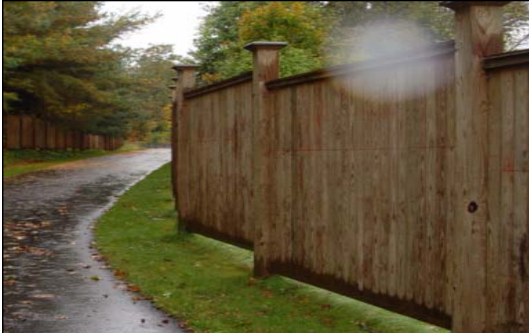
Figure 17: Wood Privacy Fence/Wall
