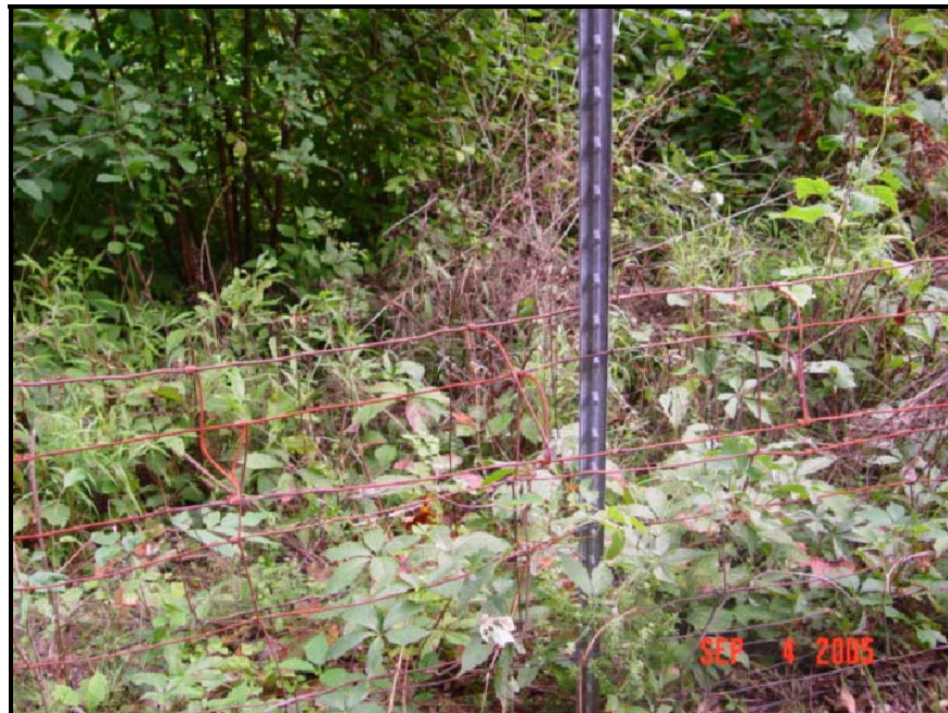
Figure 47: Barre - Deteriorated Wire Mesh fencing
