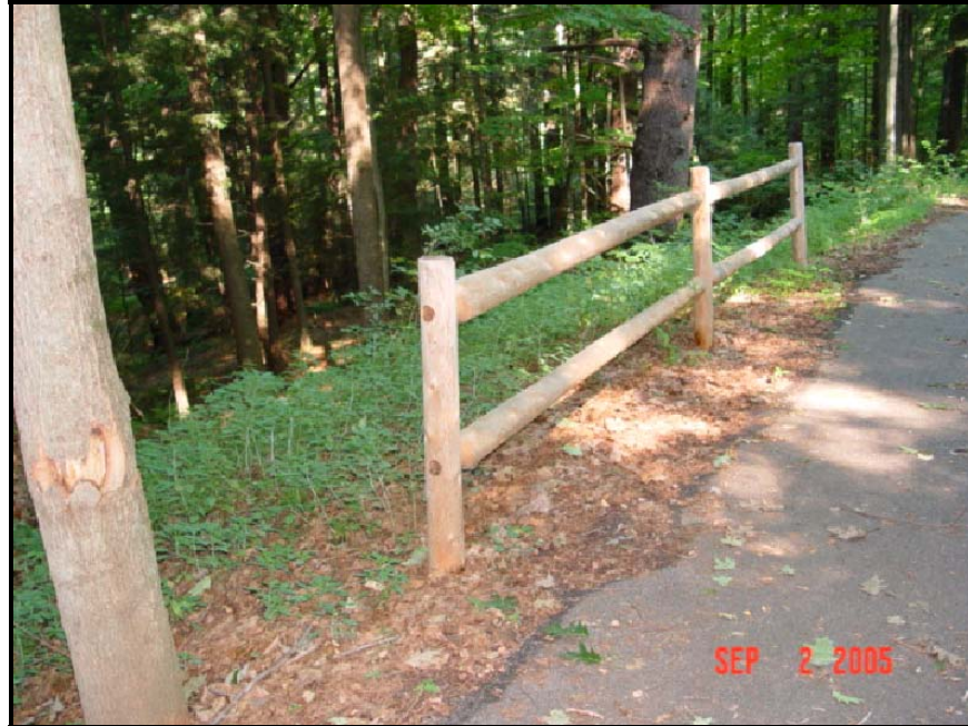
Figure 49: South Burlington - Inconsistent Use of Fencing
