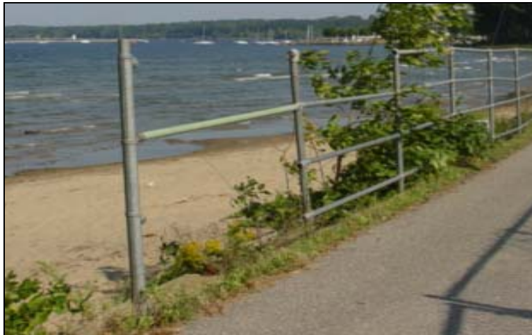
Figure 21: Metal Pipe Fence
