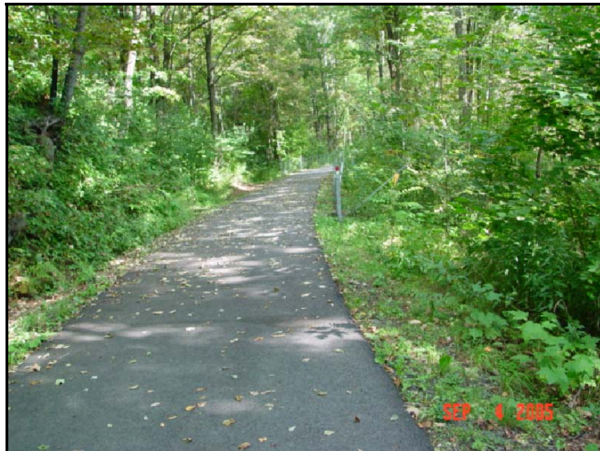
Figure 37: Barre -Vegetation Debris
