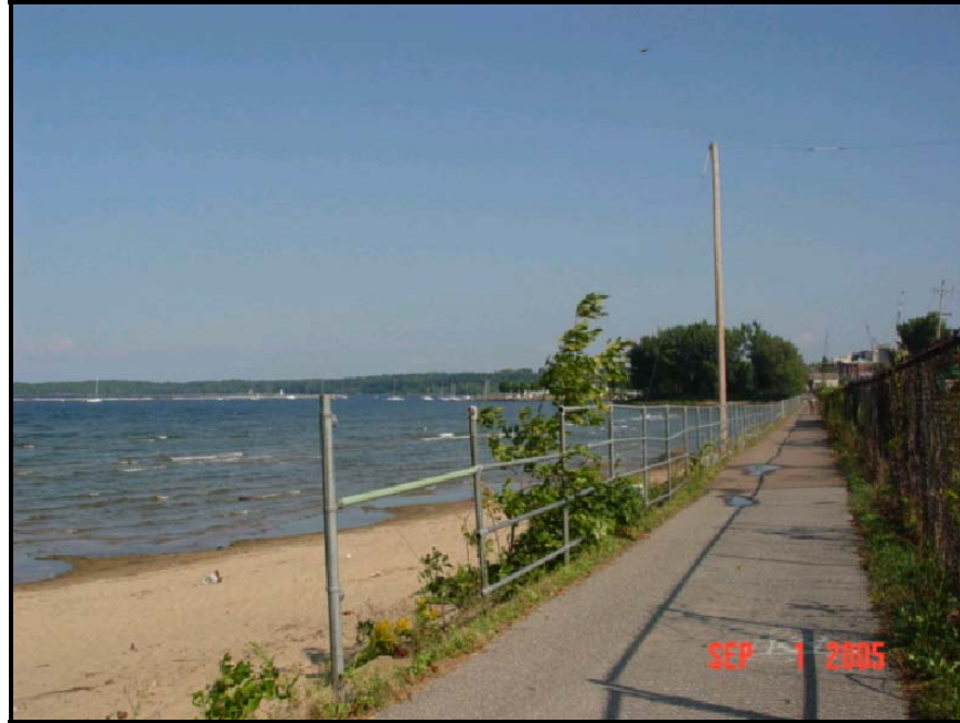
Figure 48: Burlington Waterfront - Deteriorating Pipe Fence
