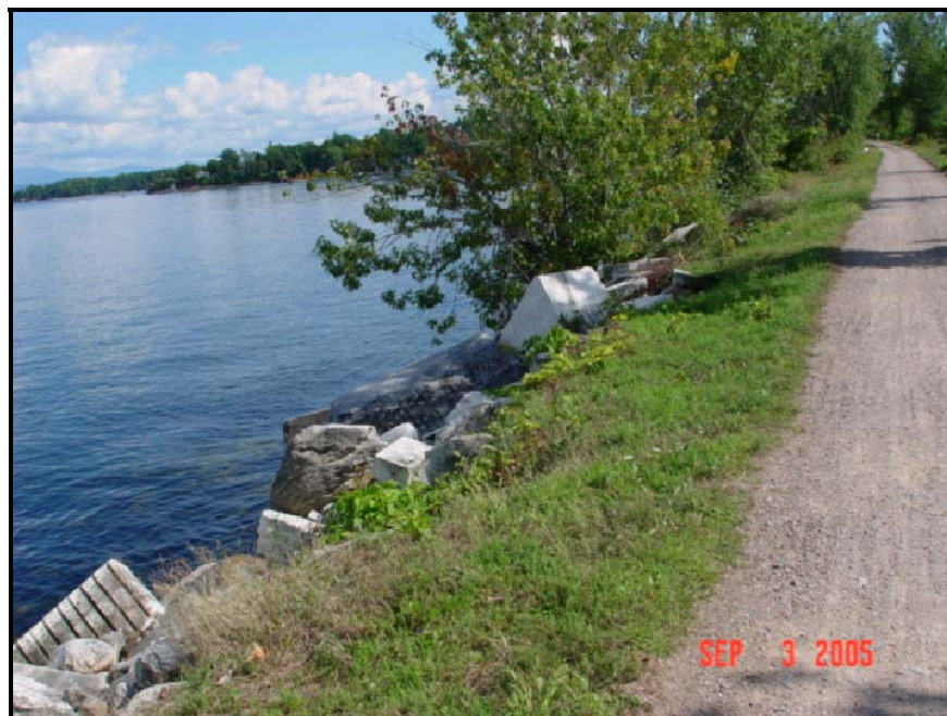
Figure 32: Colchester Causeway - Boulders at Water Body
