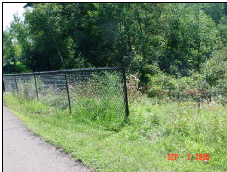
Figure 50: South Burlington - Inconsistent Use of Fencing
