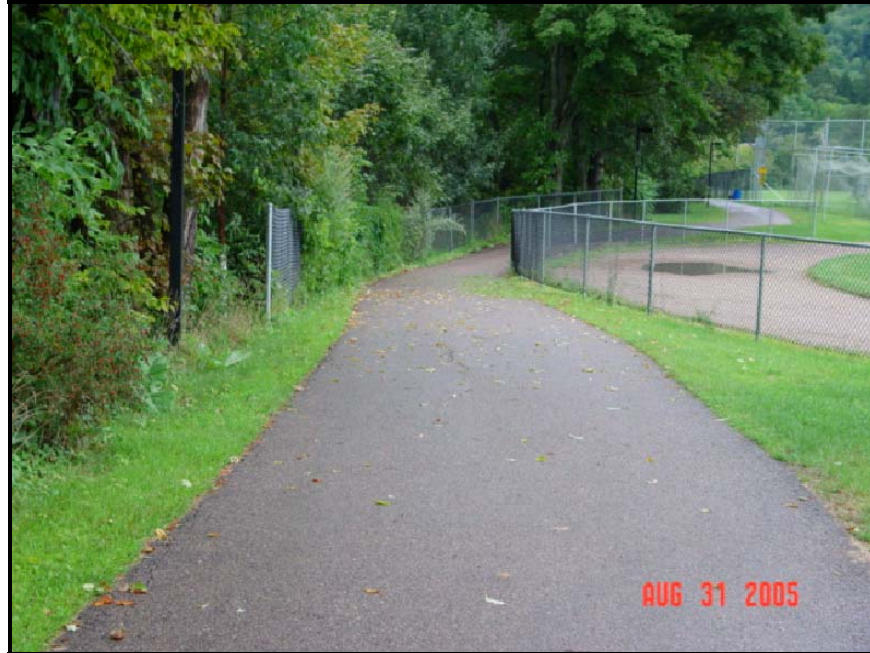
Figure 46: Montpelier Winooski - Fencing at Curve
