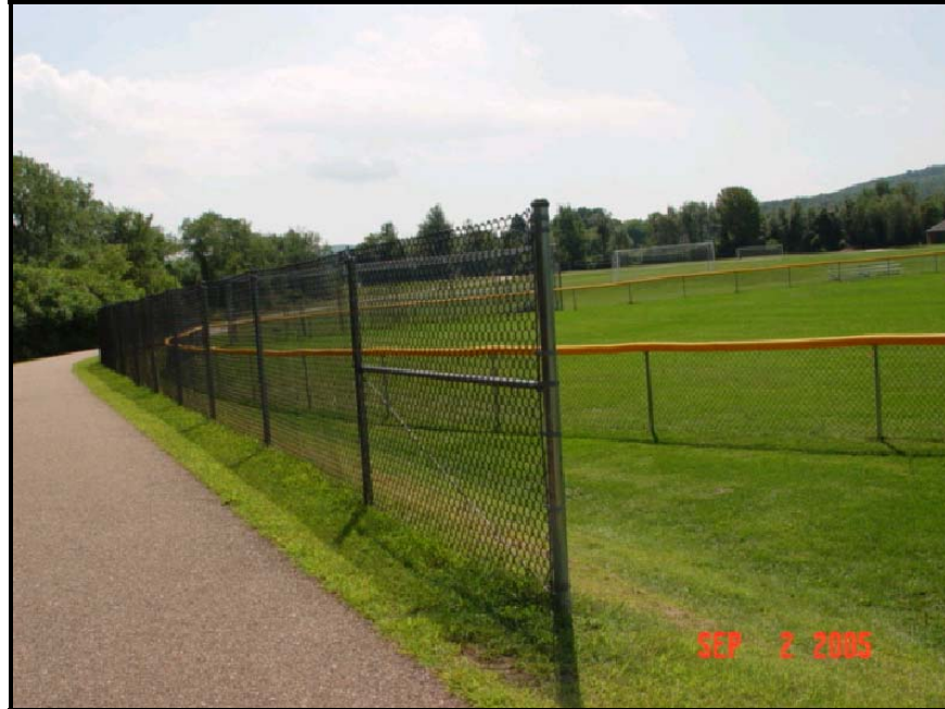
Figure 44: Williston - Chain Link Fencing at Curve
