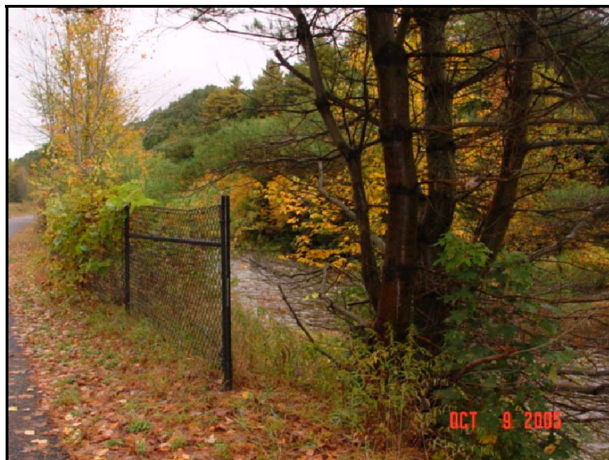
Figure 56: Toonerville - Inconsistent Use of Fencing
