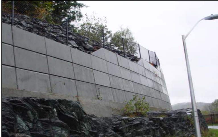
Figure 22: High Concrete Wall with Chain Link Fence
