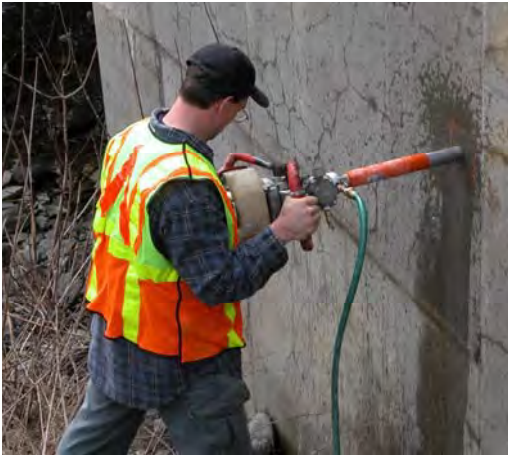
Figure 2 Coring vertical surface. Figure 3 Coring horizontal surface.
