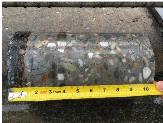
Figure 38: Core at Location 3 (L3) from Area 3 on Bridge 76.
