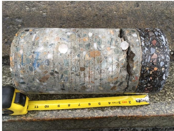
Figure 29: Core at Location 2 (L2) from Area 2 on Bridge 76.
