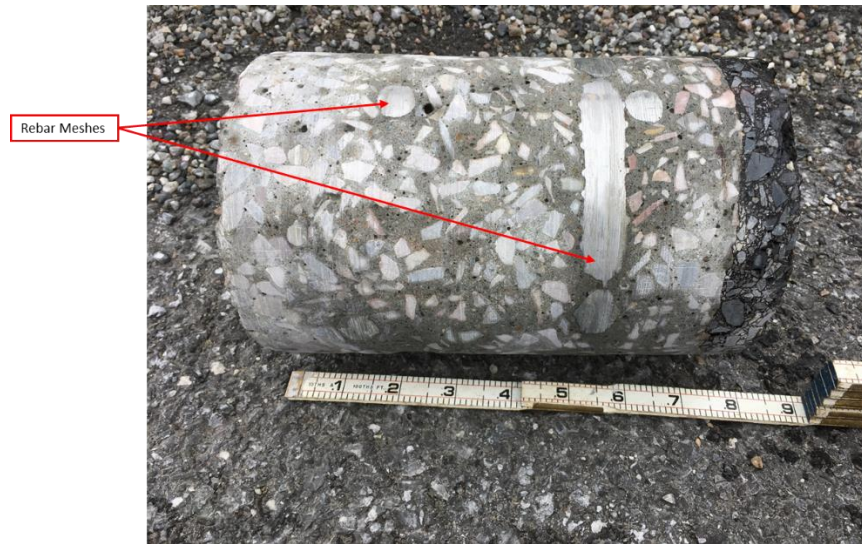
Figure 19: Area 2, L3 Core on Bridge 77. Rebar Meshes were Present.
