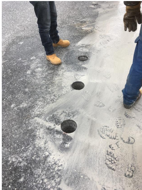
Figure 16: Area 2 Coring Holes on Bridge 77.
