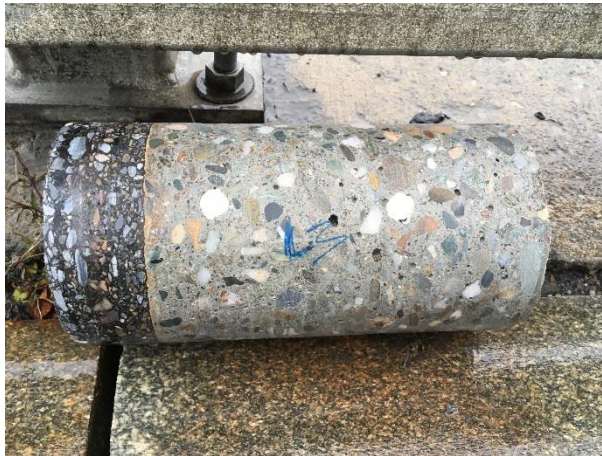
Figure 32: Core at Location 3 (L3) from Area 2 on Bridge 76.
