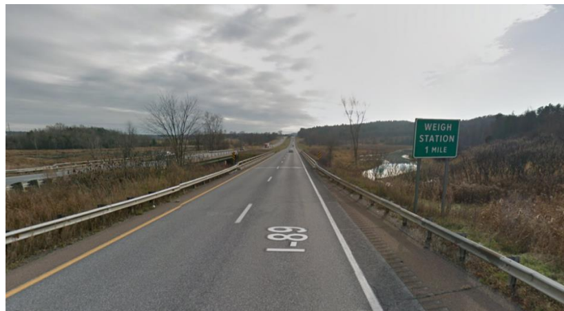
Figure 2: Street View of Bridge 77 on I-89 at MM 96.566 (Google Maps)
