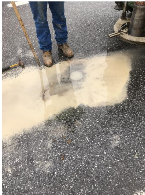
Figure 30: Core Hole at Area 2 on Bridge 76.
