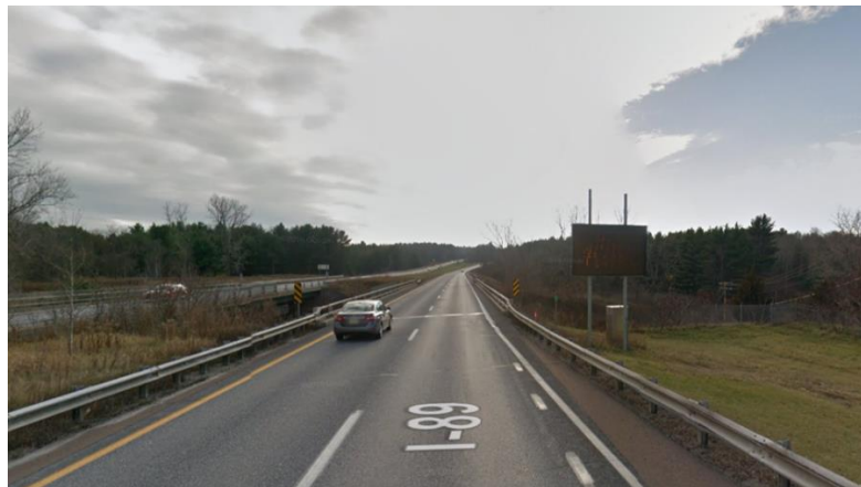
Figure 25: Street View of Bridge 77 on I-89 at MM 96.566 (Google Maps)
