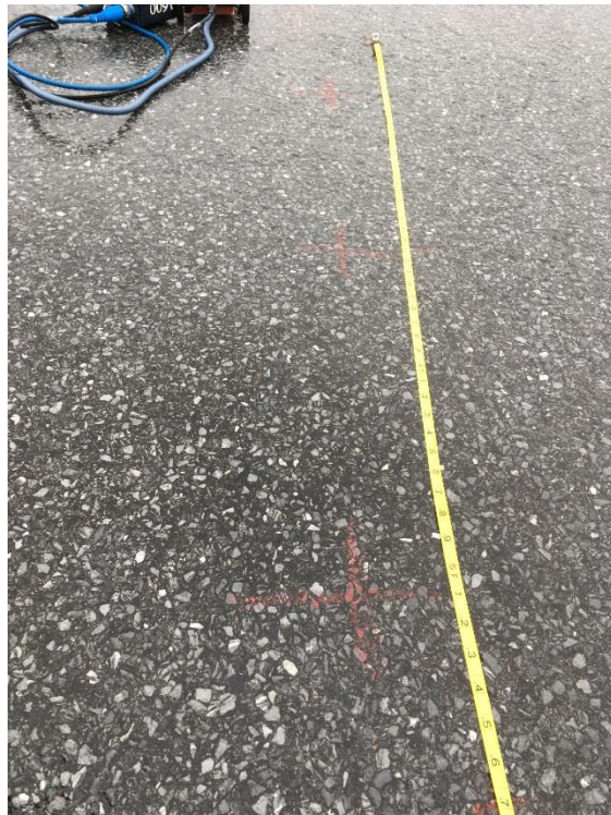
Figure 36: GPR Scan Path (Parallel to Roadway) on Bridge 76 at Area 3.
