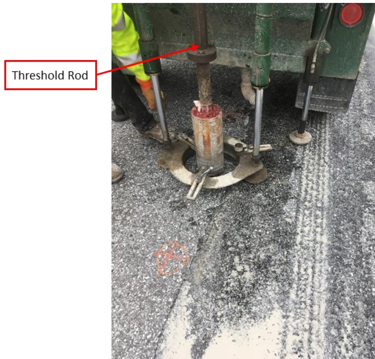
Figure 15: Drilling 6in Cores at Area 2 on Bridge 77.
