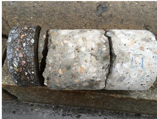
Figure 31: Core at Location 1 (L1) from Area 2 on Bridge 76.
