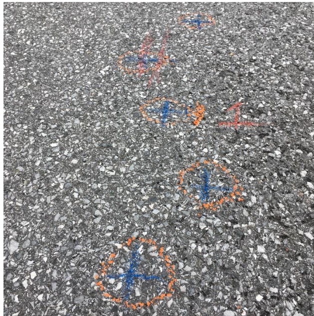
Figure 5: Close-up of Area 1 Initial Drilling Layout.
