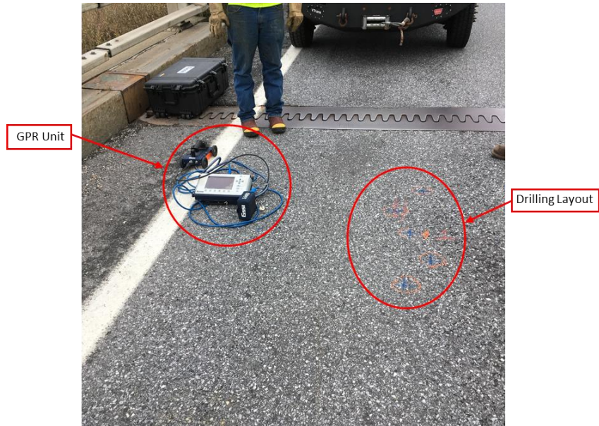
Figure 4: Area 1 Initial Drilling Layout and Handheld GSSI GPR Unit.
