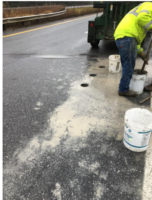
Figure 39: Core Holes on Bridge 76 at Area 3
