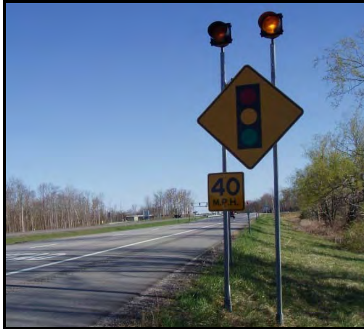
Figure 11 Typical Advanced Warning Flasher (AWF)
