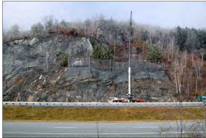
Figure 15 Hoisting Panels onto Steel Posts and Steel Support Ropes.
