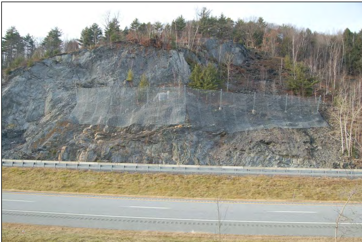
Figure 1 Photograph of Hybrid Barrier/Drape Installation, I-91, Fairlee, Vermont.
