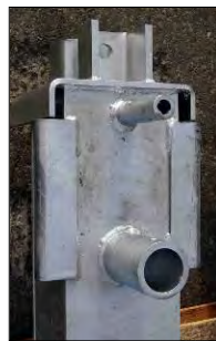
Figure 10 Close-up of the Top of Steel Post.
