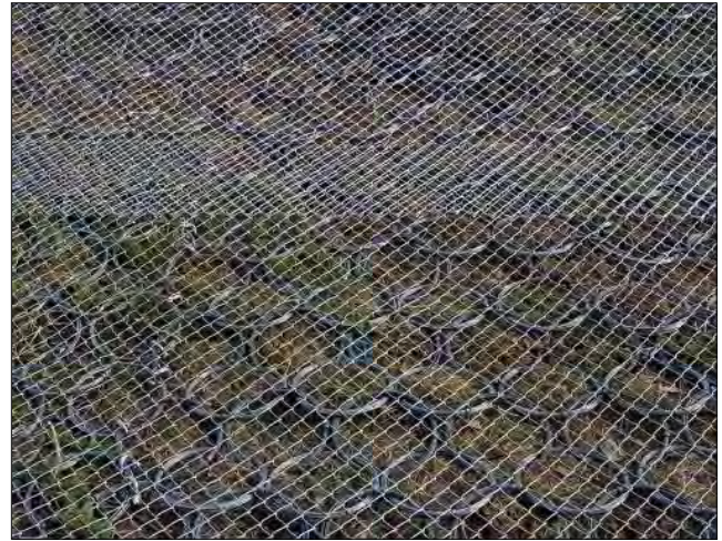
Figure 12 Connecting Chain-Link Mesh to Ring Nets.
