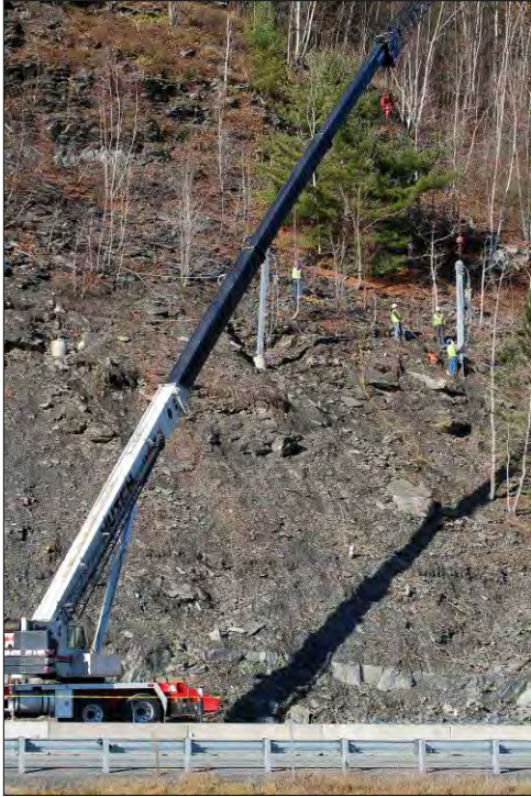
Figure 14 Placing Steel Posts.
