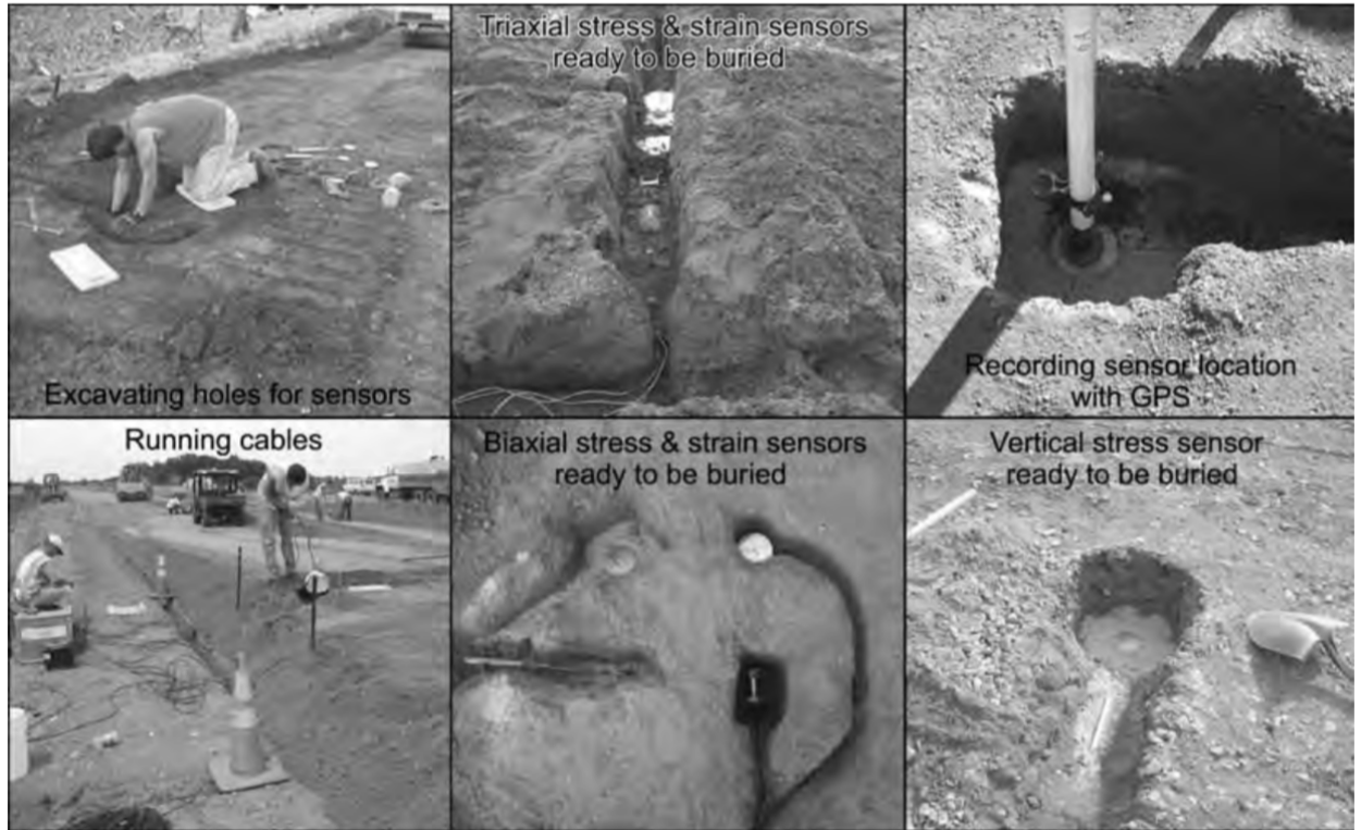
Figure 9. Photographs showing different stress/strain sensors employed to capture the soil behavior (Source: NCHRP report 676 [Mooney et al., 2010])
