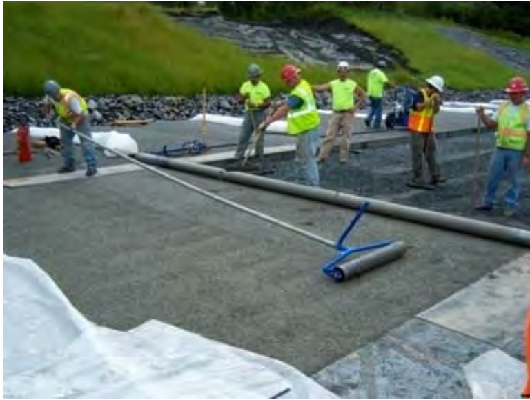
Figure 2.3: Finishing with Roller Screed and Steel Roller
