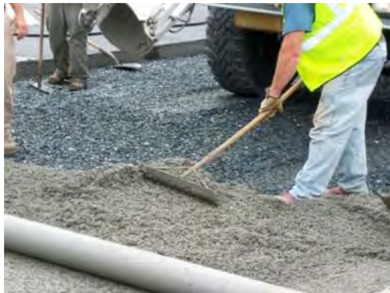
Figure 2.2: Placing Porous Concrete Material
