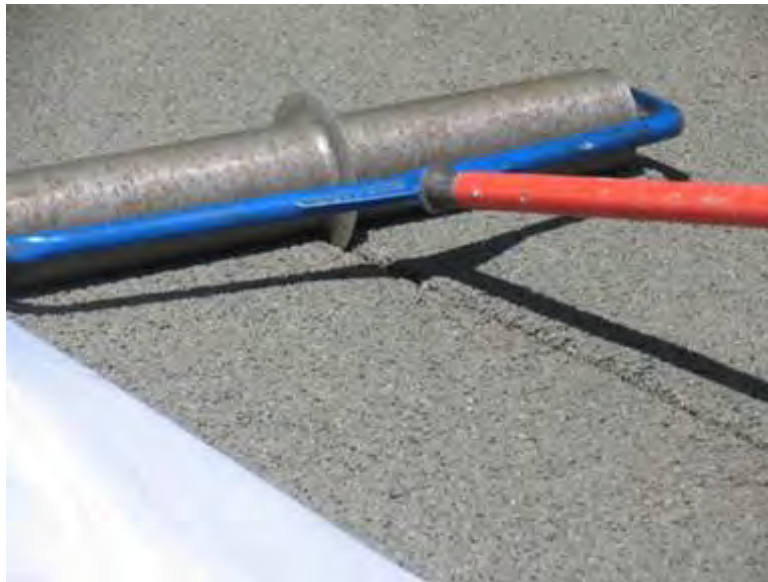
Figure 2.4: Control Joint being Rolled In
