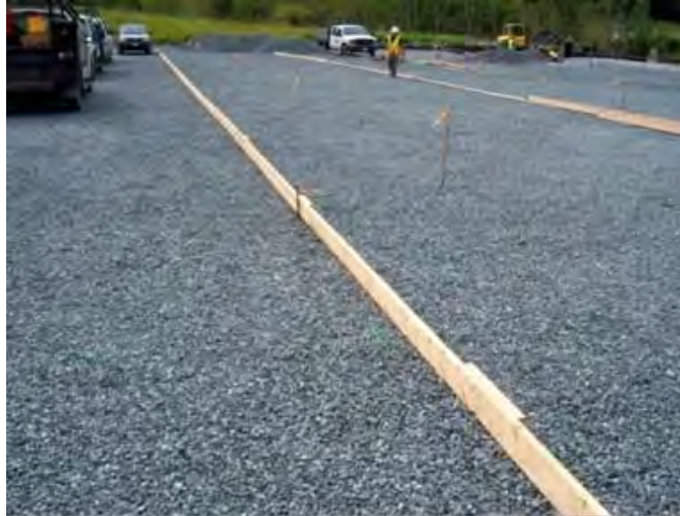
Figure 2.1: Gravel Subbase with Wooden Forms Placed
