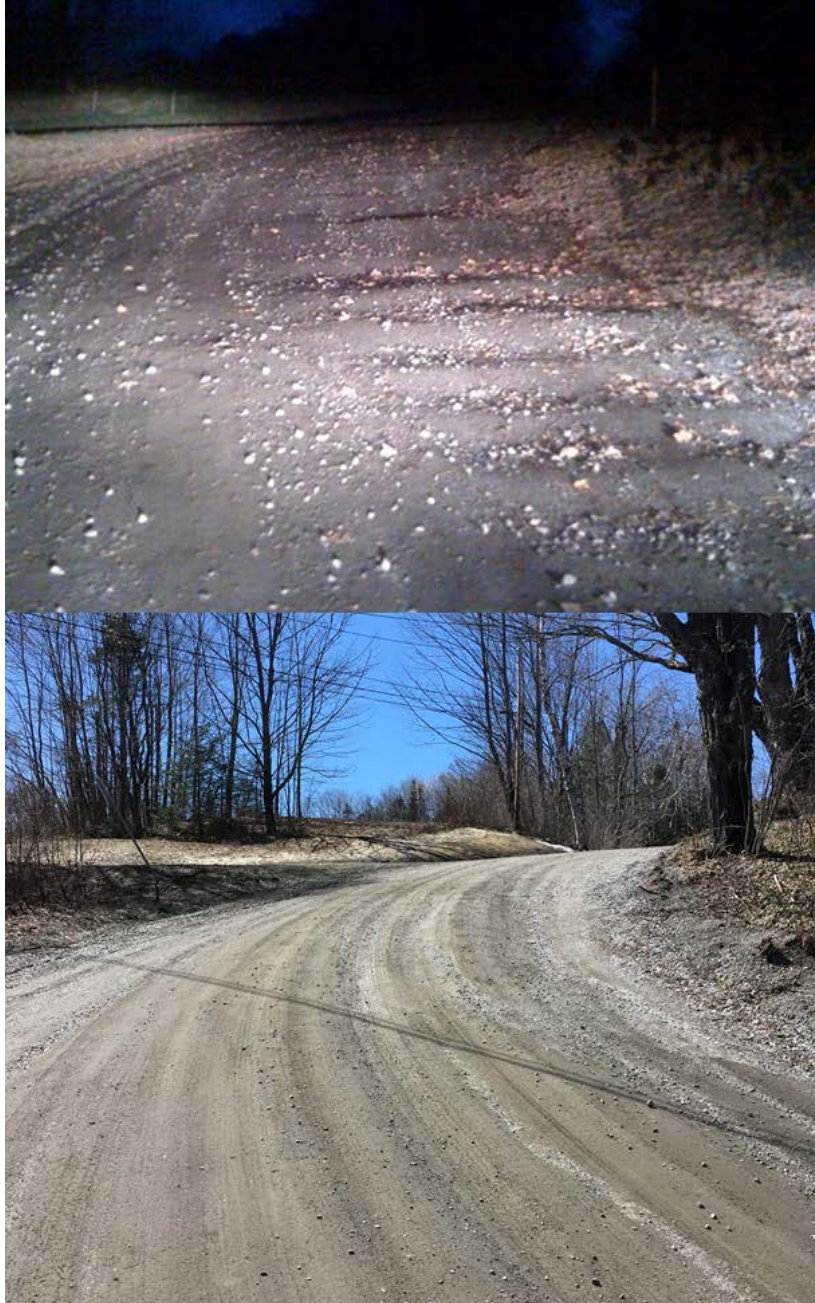
Figure 2: Intersection with West Street at VT 65 Mile Marker 2.5. Photo Comparison between 10/26/16 Site Visit (Top) and 4/14/17 Site Visit (Bottom)
