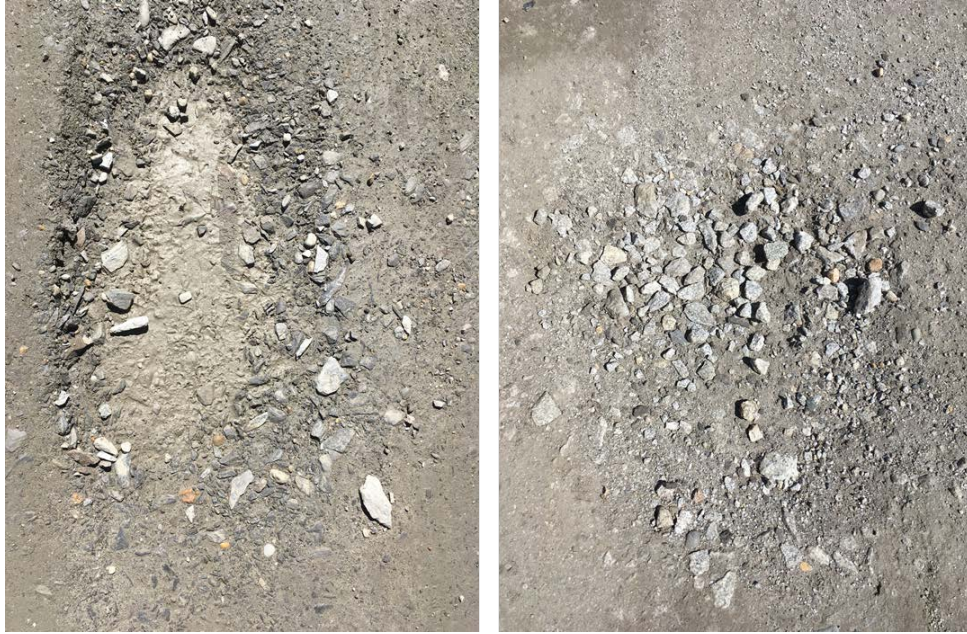
Figure 8: Bear Hill Rd Pothole Near Intersection with VT 65. Road has no RAS, aggregate is more irregular (Left). Pothole on VT 65 East of Bear Hill Rd near Mile Marker 2.1. Road has RAS, aggregate is more cubic (Right). Photos taken during 4/14/17 Site Visit.
