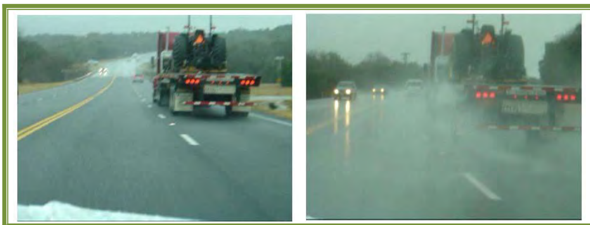
Open-graded friction course (left) compared with conventional pavement (right) (Barrett & Shaw, 2006, used with permission)
