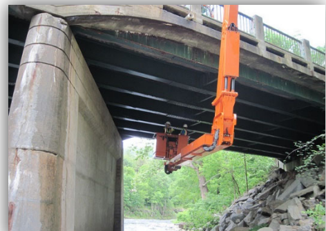
VTrans bridge inspectors at work.
