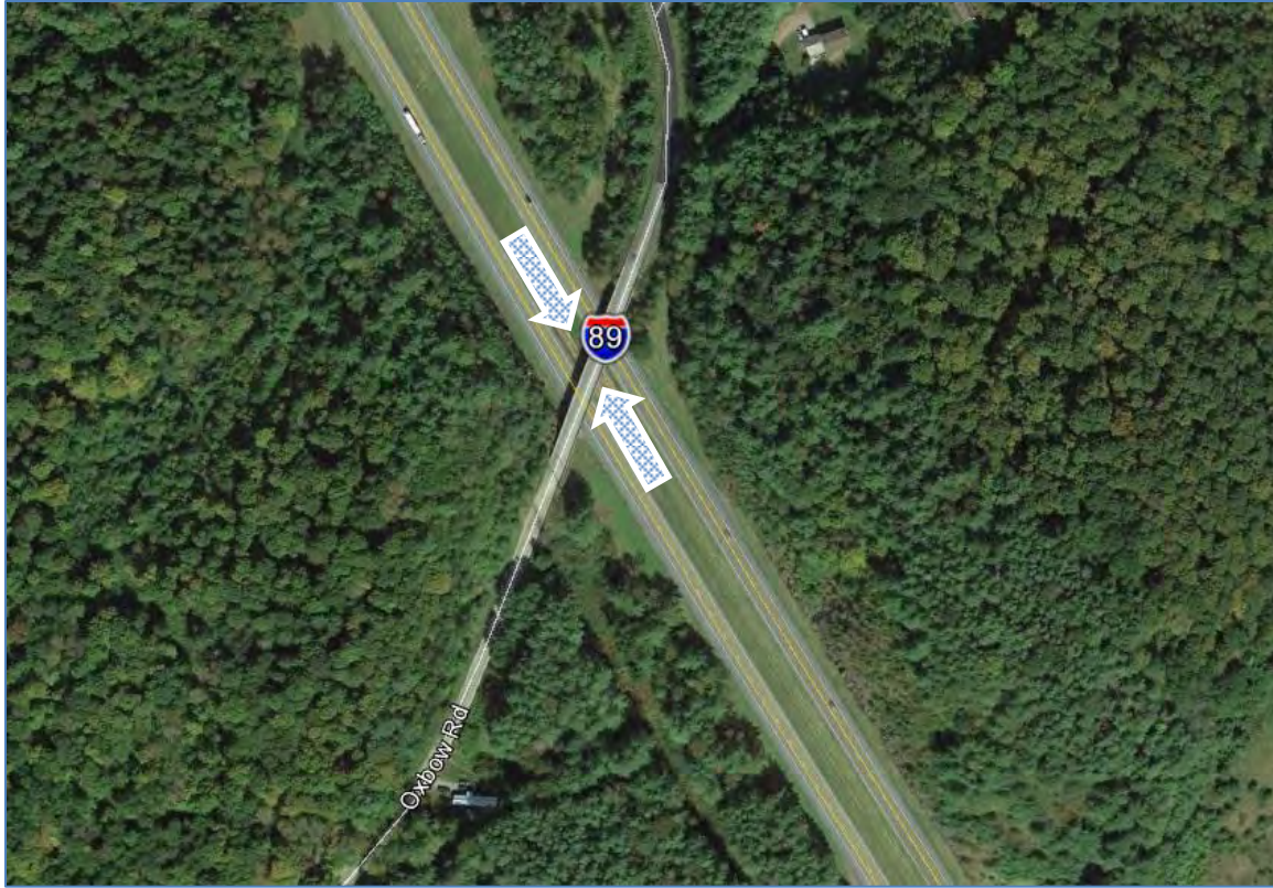
Figure 9 Aerial View of the Vicinity of the Locally-optimal Royalton SSF
