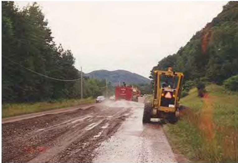
Figure 4 Water application during RSB construction
