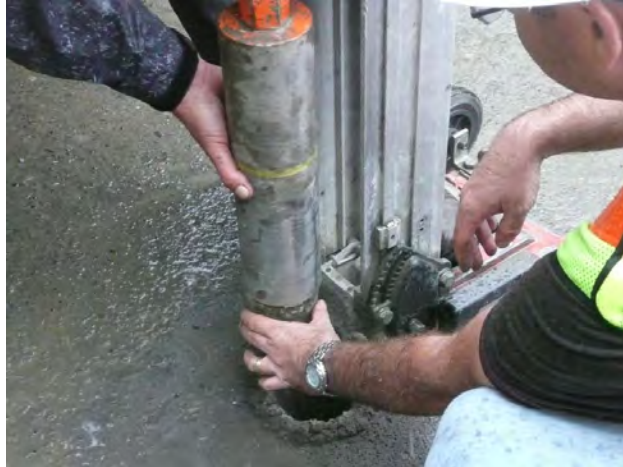
Figure 6 A typical 4” core being drilled and extracted on a project.
