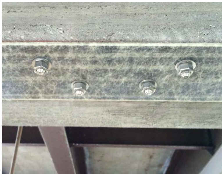
Figure 11 Completed Pattern of Bolts (VTrans 2014)
