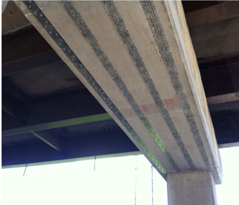
Figure 12 Completed FRP Installation (VTrans 2014)
