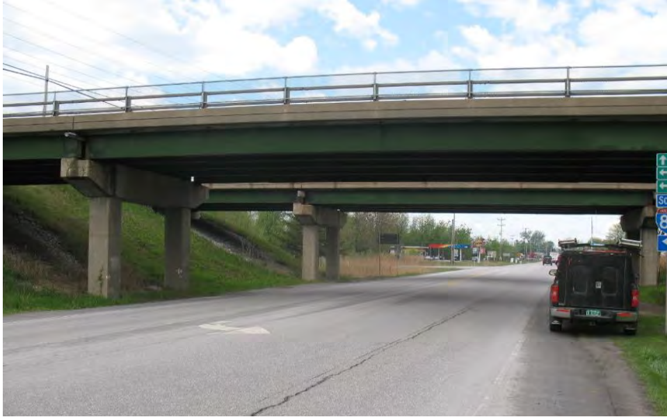
Figure 2 Project site – I-89 Bridge 98 over VT 78 in Swanton (VTrans 2010)
