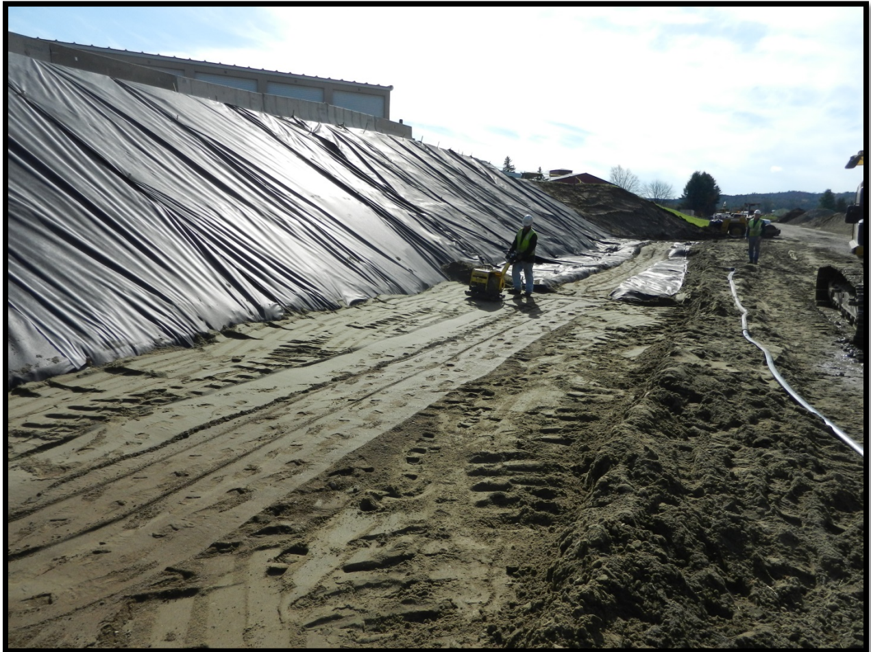
Figure 2: Geotextile fabric installed as a grade separator & leveling pad construction
