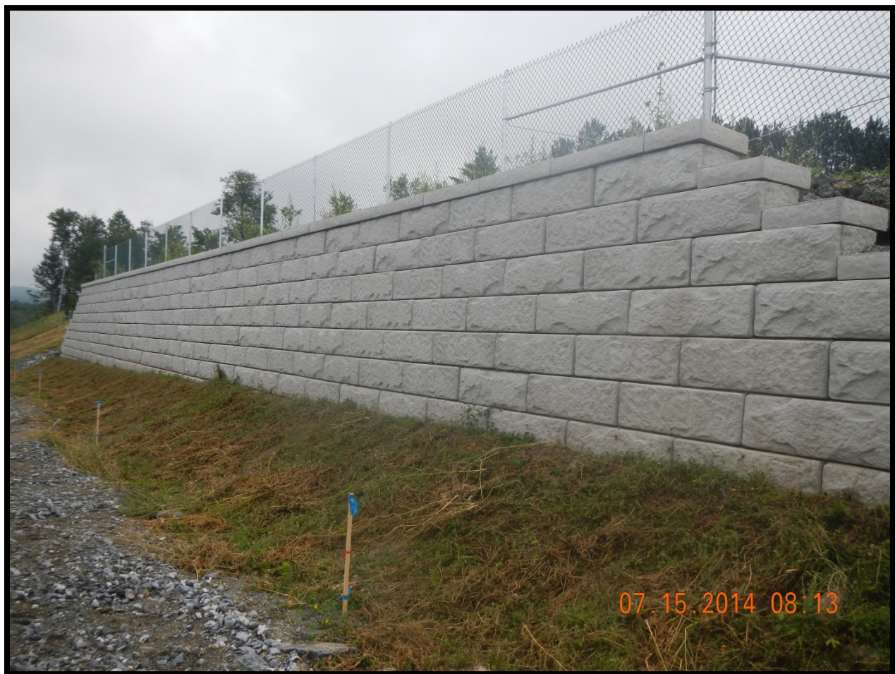
Figure 7: Completed ReCon retaining wall
