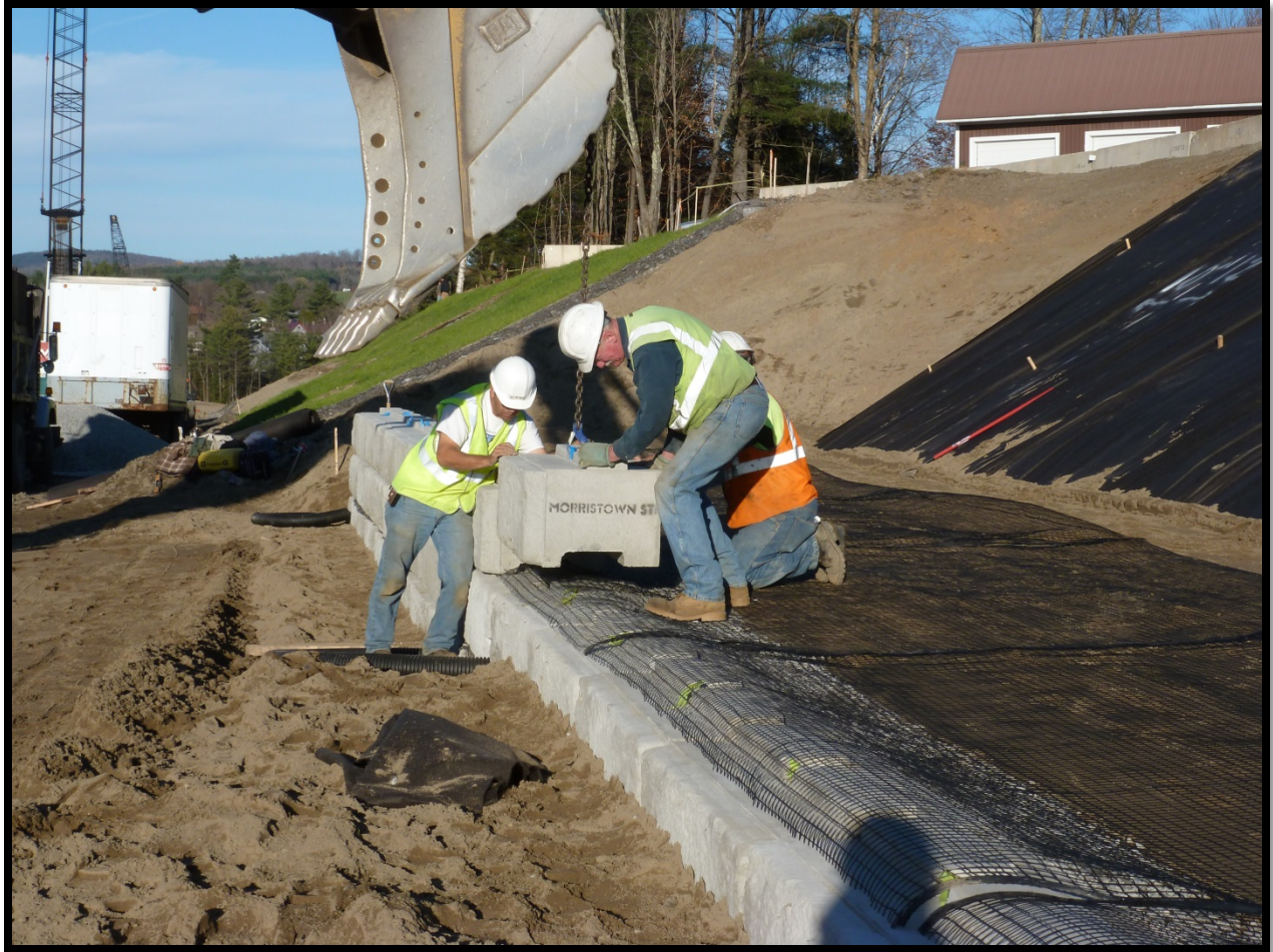
Figure 6: Installation of a row of blocks
