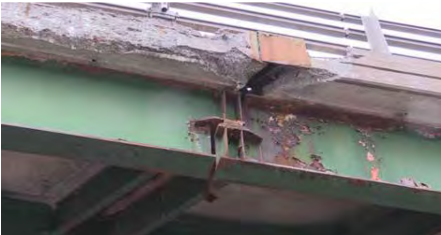
HARTFORD. One of the I-91 bridges.
