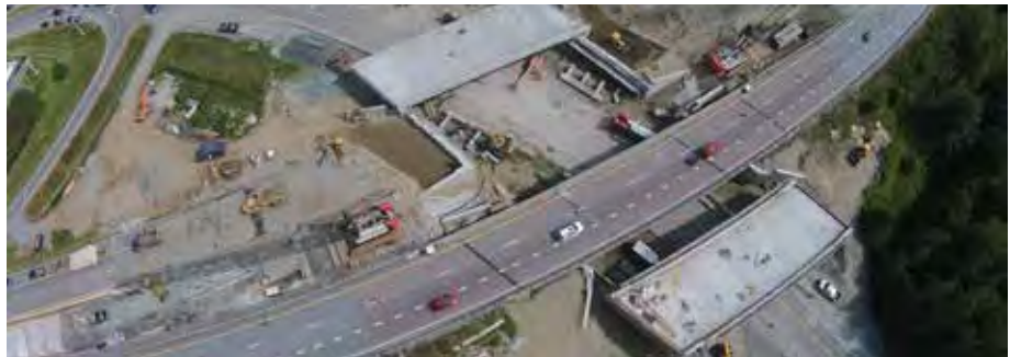
HARTFORD. Using slide-in construction methods, two bridges on I-91 were replaced over two weekends in August.
