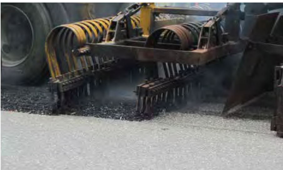
Hot recycled in place pavement.
