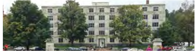
MONTPELIER. DMV main office.
