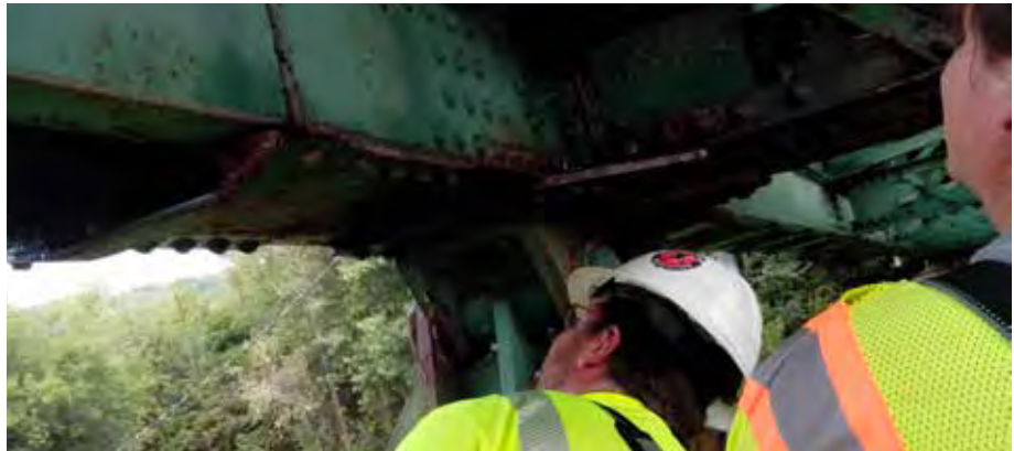
HARTFORD. Inspectors examine Bridge 7 across the White River.
