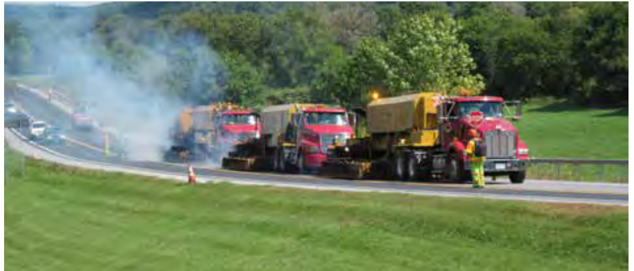
WAITSFIELD / MORETOWN. Paving project.
