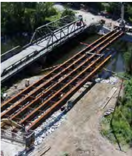
RUTLAND. River Street town highway bridge.
