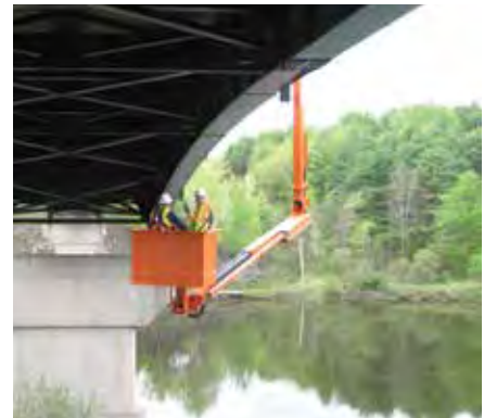
MILTON. Inspecting the I-89 bridges over the Lamoille River.
