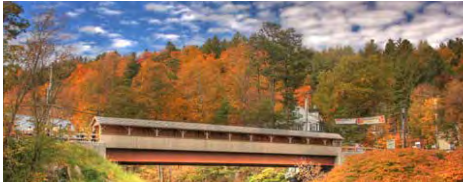
STOWE. Bridge 2, located in the heart of Stowe Village along VT 108, was replaced using innovative construction techniques during a 40 day closure in April and May of 2015.
