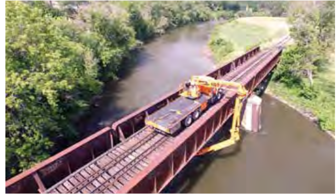
MONTPELIER. VTrans Rail Bridge Inspection Team operating the brand new Aspen Aerials A30 "Snooper" truck at bridge 305 on the Washington County Railroad this Spring.
