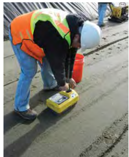
Testing material density.
