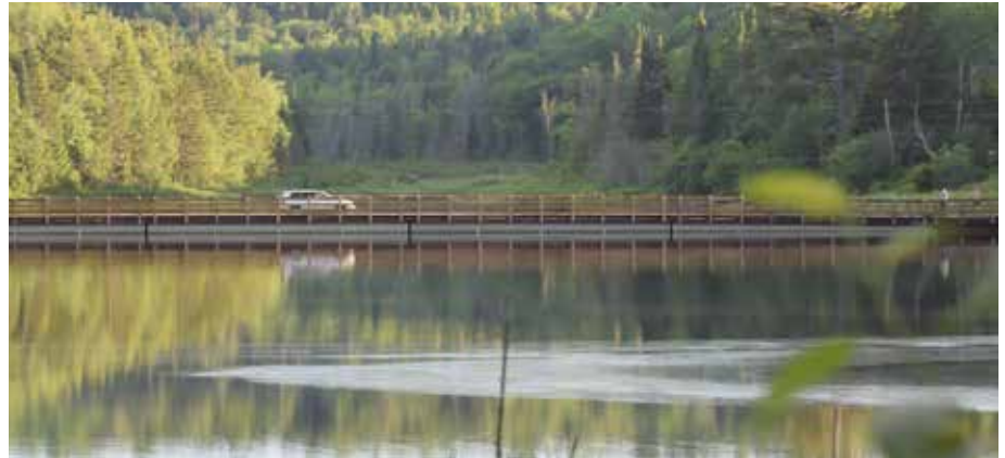
BROOKFIELD. The Floating Bridge is one of only three such bridges in the United States.
