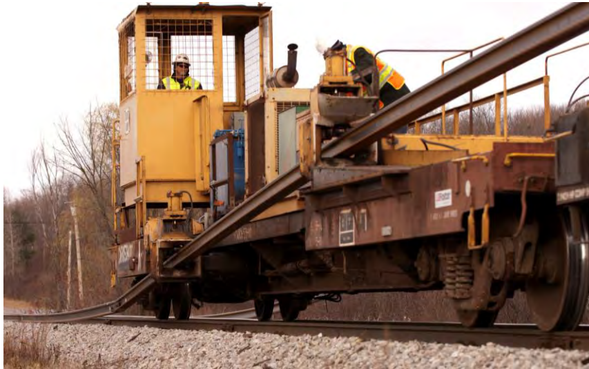
Figure 7.3 New England Central Railroad Rail Replacement Project, 2011
