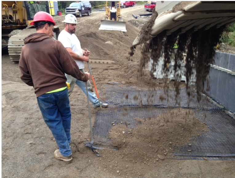
Figure 12: Applying subbase material over geotextile layers (1)
