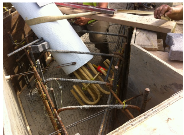
Figure 9: Anchorage reinforcement of the tubes
