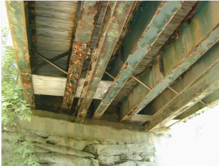
Figure 5: The underside of bridge showing the added beams
