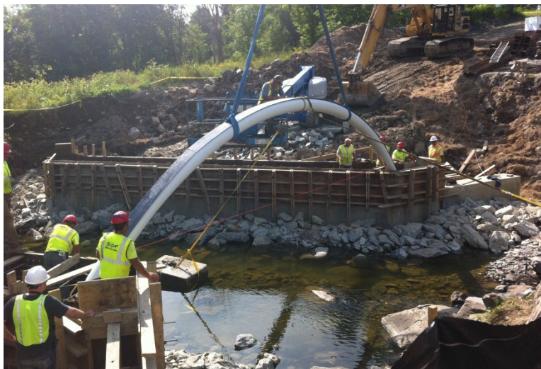
Figure 8: Installation of the first tube
