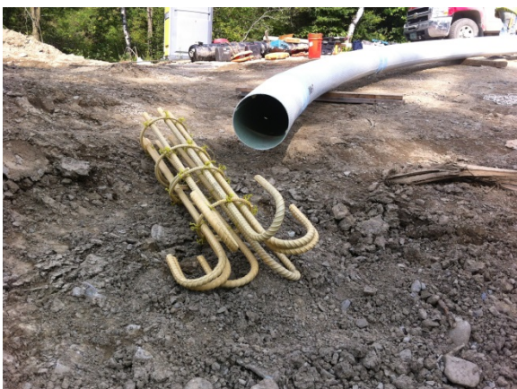
Figure 9: Anchorage reinforcement of the tubes
