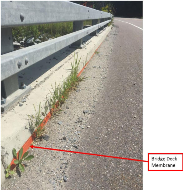
Figure 18: Bridge deck membrane (August 15 ,2017)
