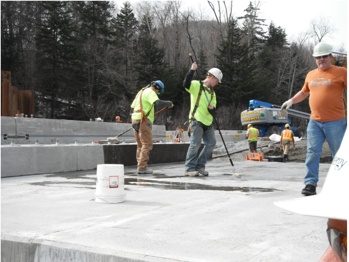
Figure 2: Installation of the BDM system, application of the primer (March 12, 2012)
