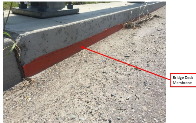
Figure 10: Bridge deck membrane (June 2, 2016)
