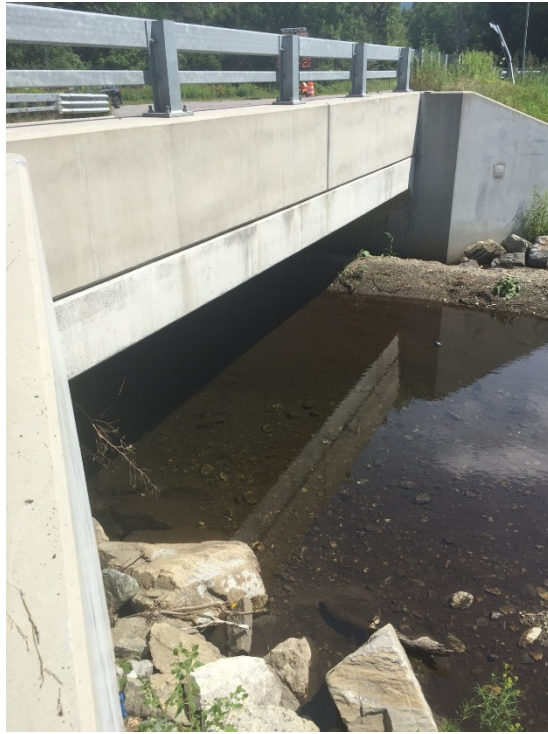
Figure 13: View of right side of bridge, facing south (August 15 ,2017)
