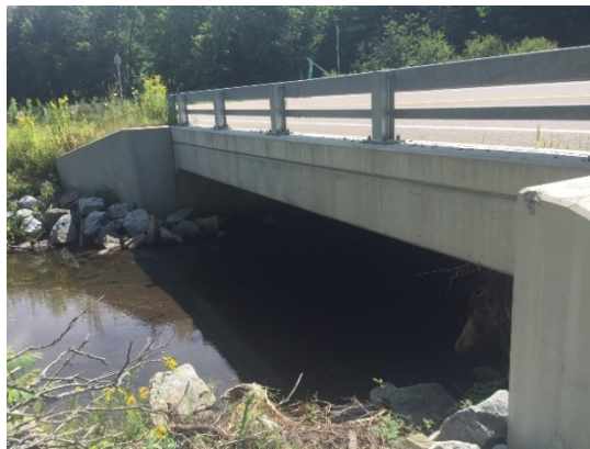
Figure 14: View of left side of bridge, facing north (August 15 ,2017)
