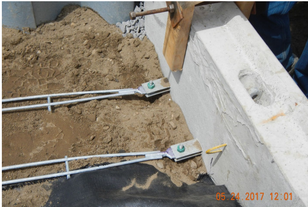
Figure 12: Reinforcing strips connected to the wall panels
