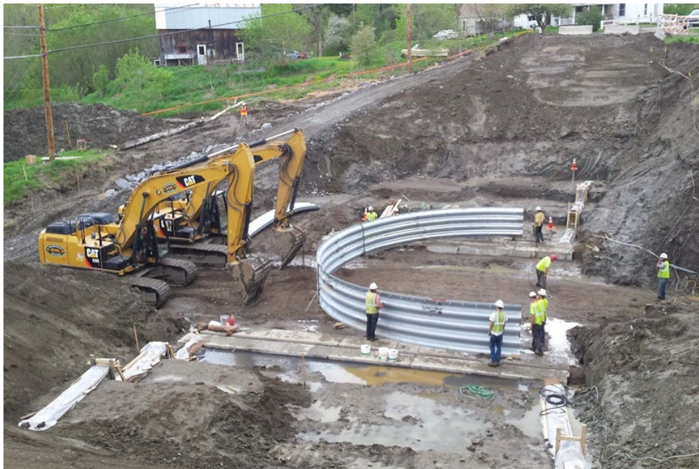
Figure 4: Constructing the first ring section
