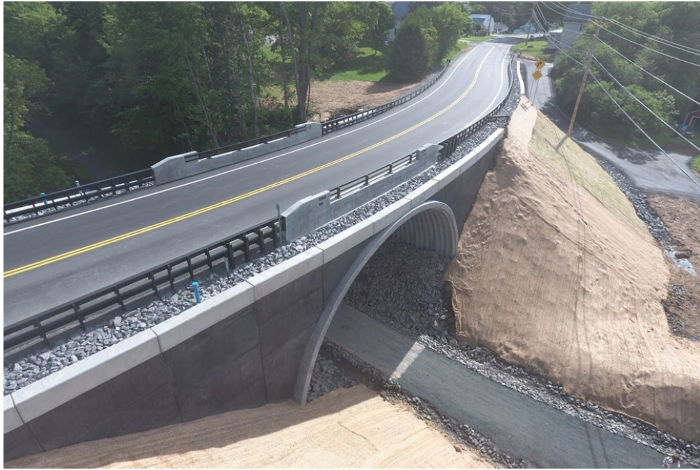
Figure 22: Completed Structure over the trail
