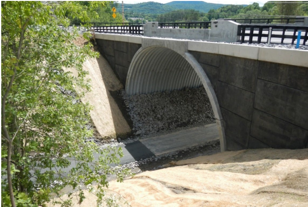
Figure 21: Completed Vist-A-Wall abutments and bridge
