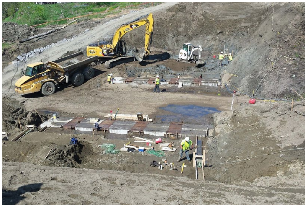
Figure 3: Curing the Closure Pour
