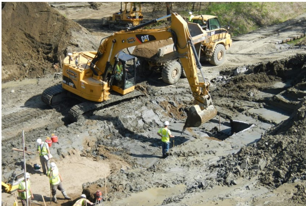
Figure 1: Excavating for the Arch Foundation
