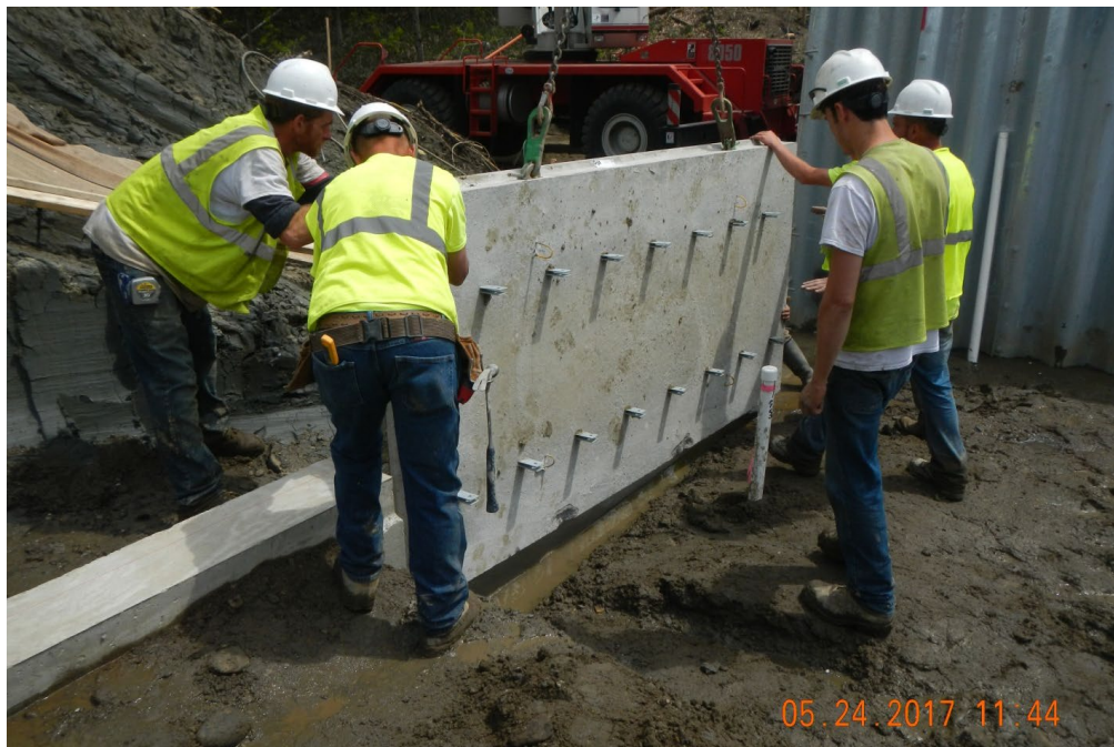
Figure 10: Example wall panel being placed on leveling pad
