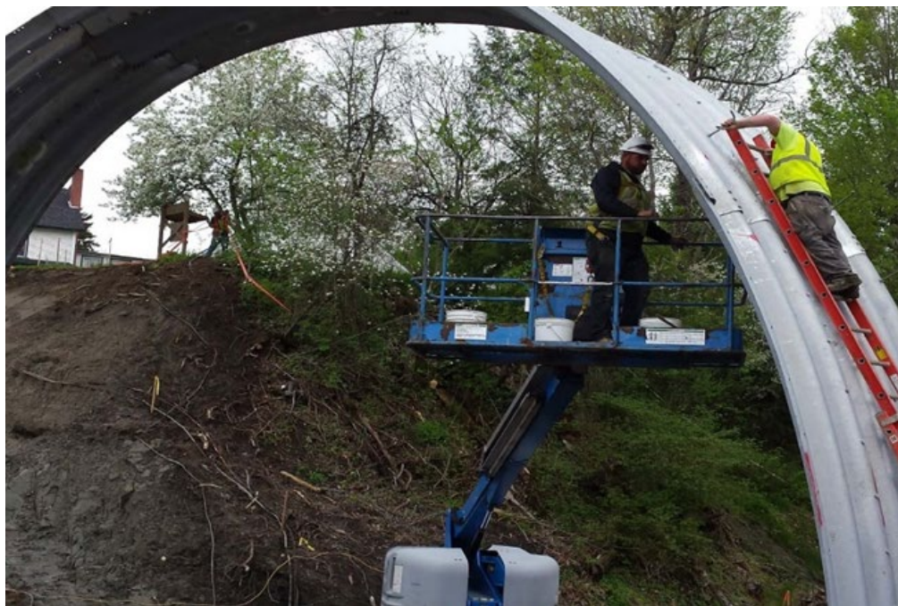
Figure 7: Contractors connecting panels with torqued arch bolts
