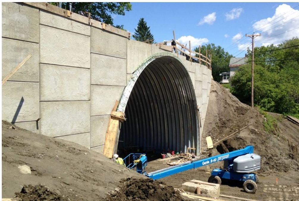
Figure 9: Arch Collar Formwork in Construction
