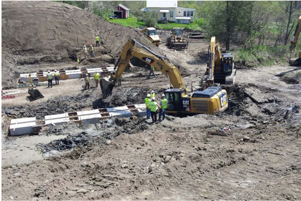
Figure 2: Arch Foundation Elements Ready for the Closure Pour
