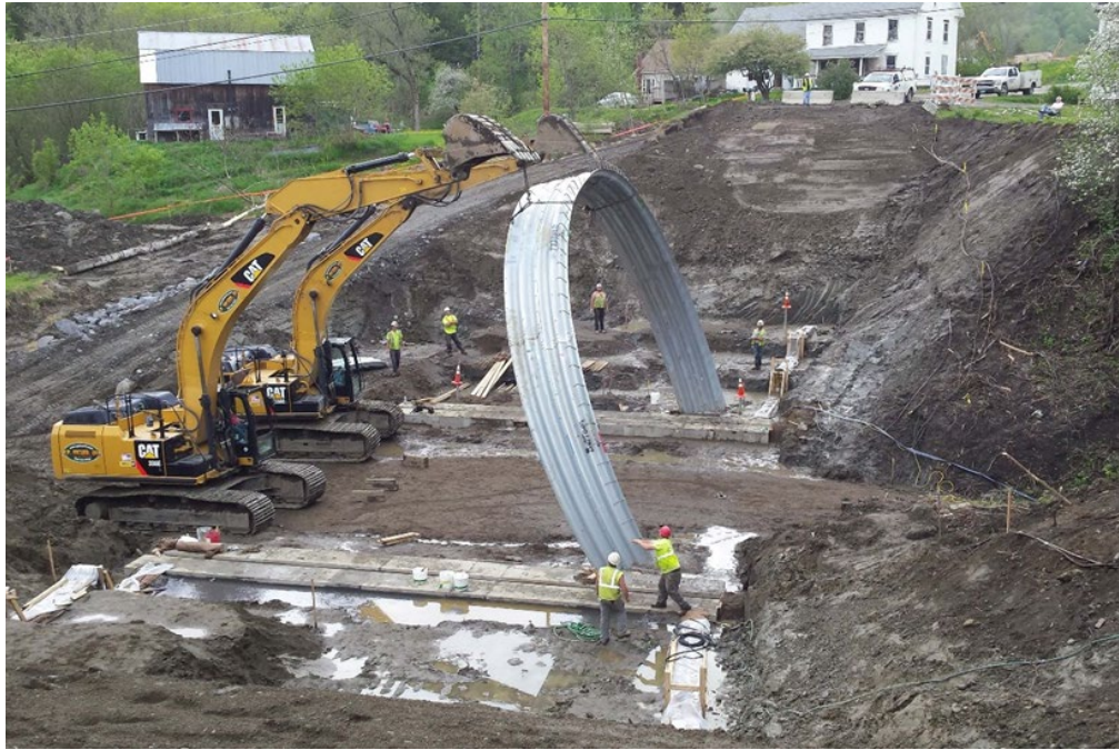
Figure 5: Raising the first ring section
