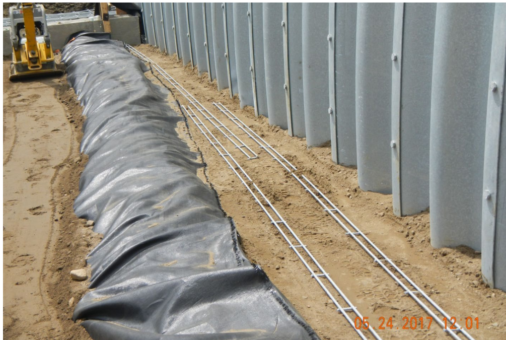
Figure 11: Steel reinforcing strips placed in backfill behind the metal arch
