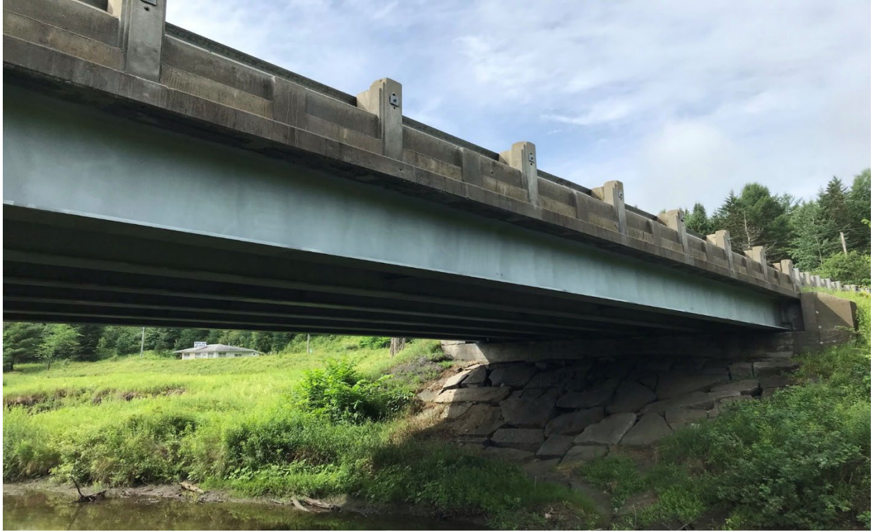
Finished Metalizing (Fascia Beam)
