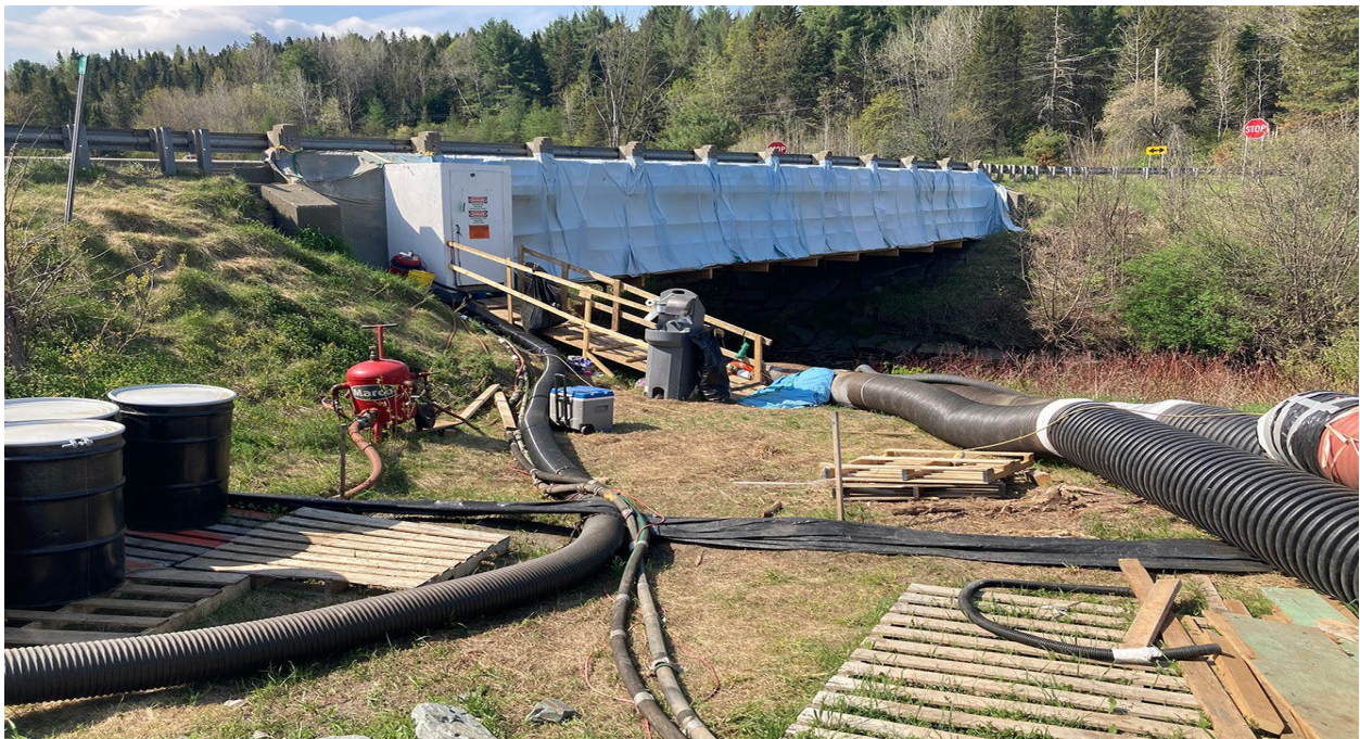
Structure Containment in Place
