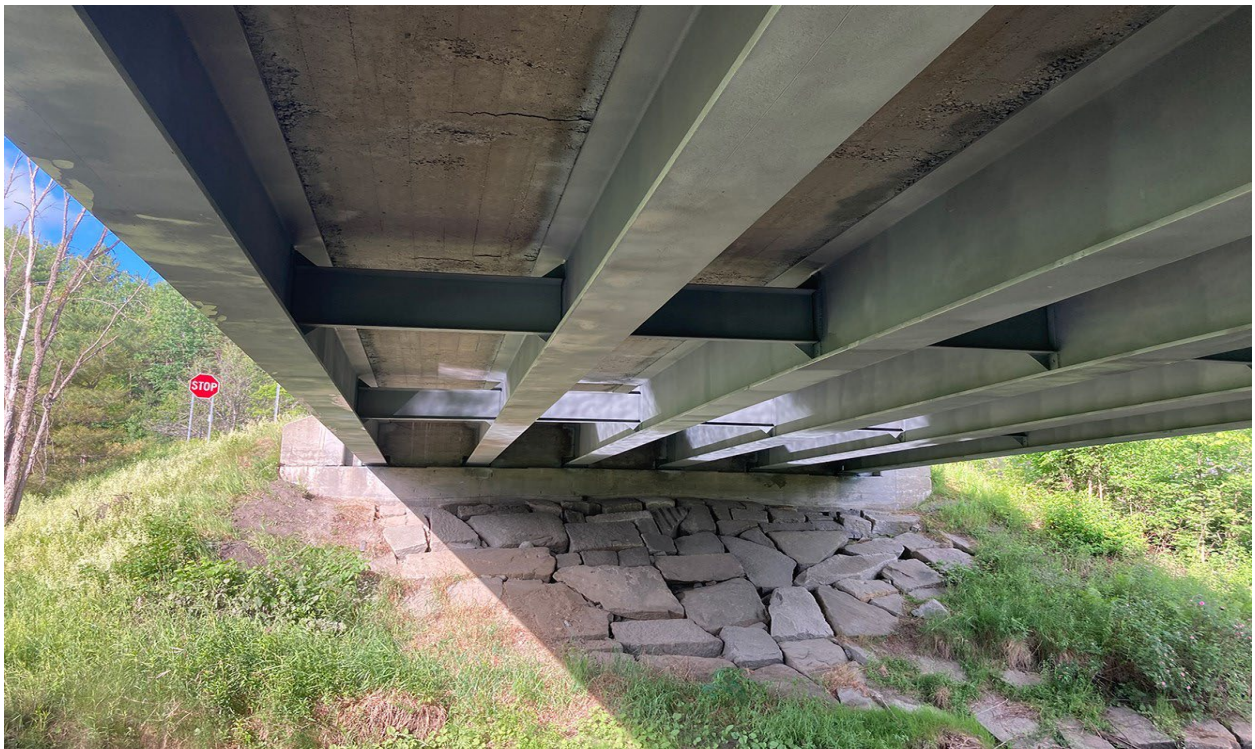
Finished Metalizing (Interior Beams)
