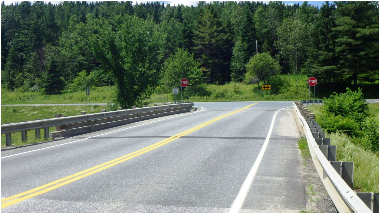
Hardwick VT 16 Br. 1 (Looking south toward VT 15)
