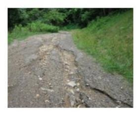
Rill Erosion = depth of 1" < 12"
