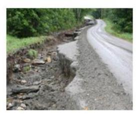
Gully Erosion = depth of 12" +
