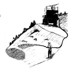
Figure 34: Hydroseeder attached to truck
