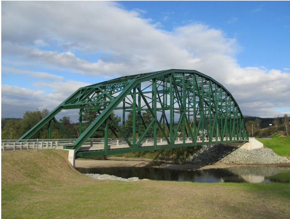
Checkered House Bridge Richmond VT
