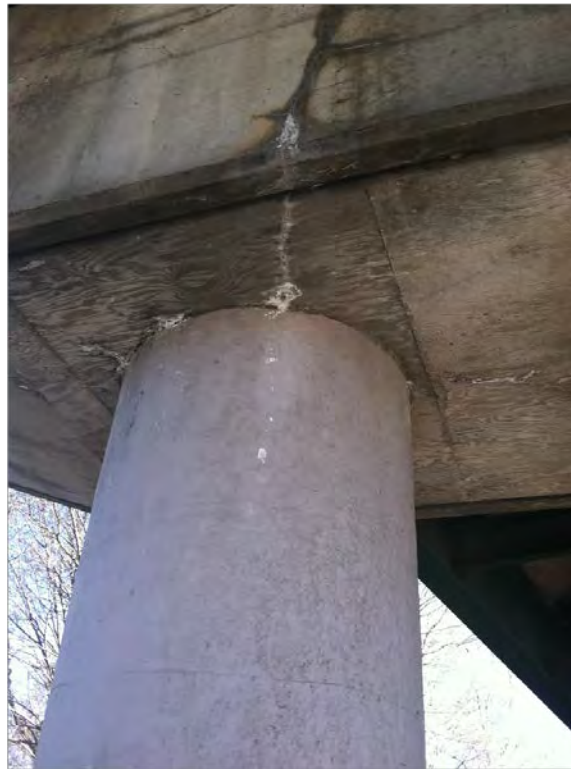
Figure 9 Chlorides leaching onto column.
