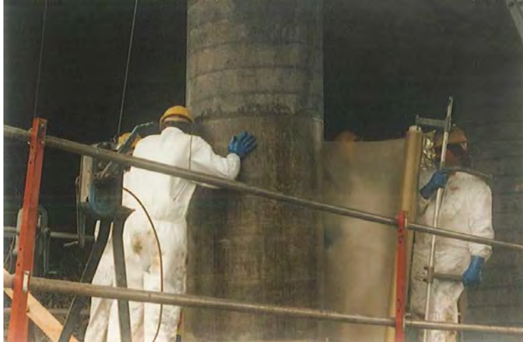
Figure 3: TYFO S Fibrwrap spindle application (1994)
