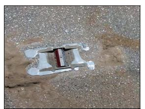
Figure 2 – Hallen Marker with Epoxy
